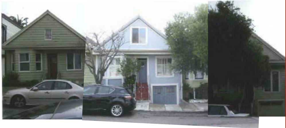
East side of Gates, North of Cortland
