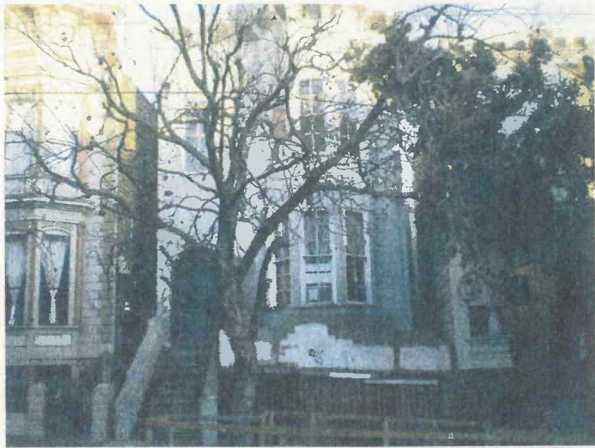
Front of subject building.
