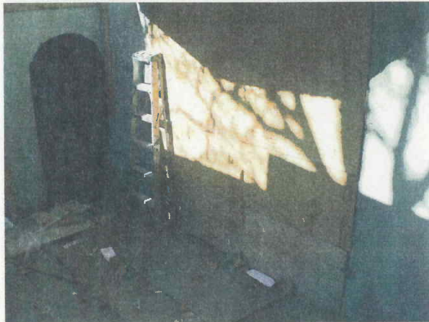
View of garage opening hidden by plywood barrier
