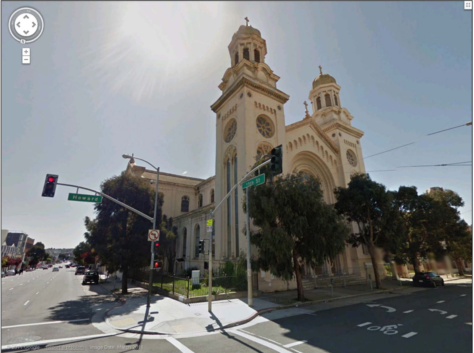
1401 Howard Street, View at southwest corner of 10 th and Howard Streets
