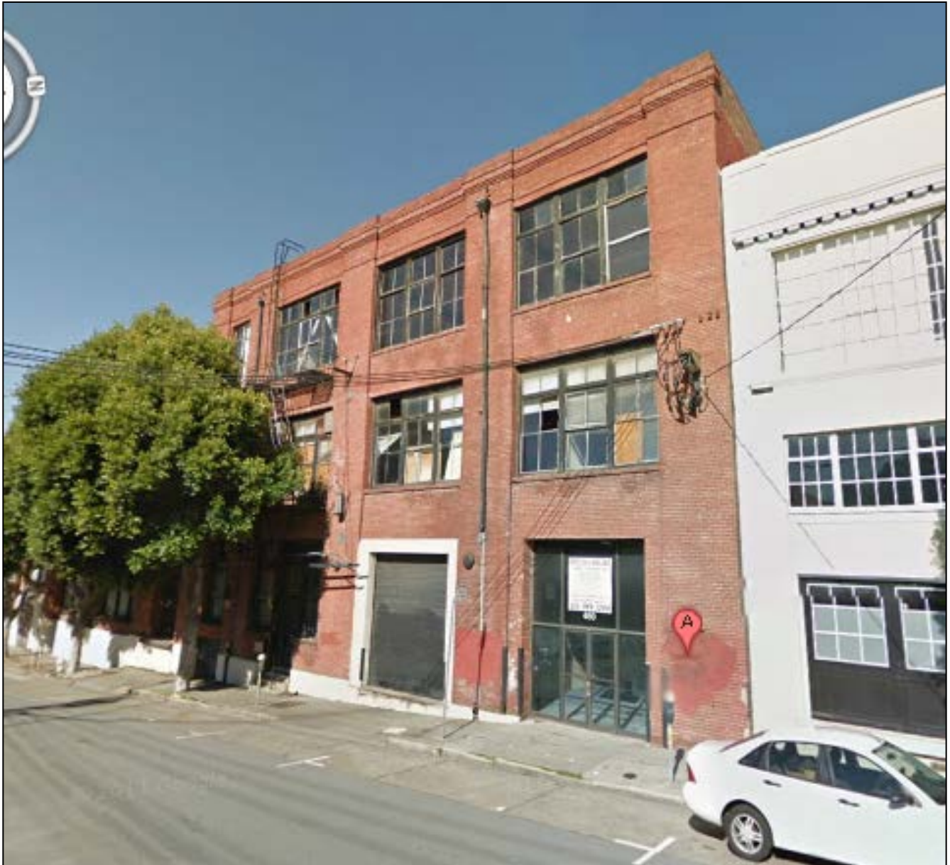
460 Bryant Street facade
