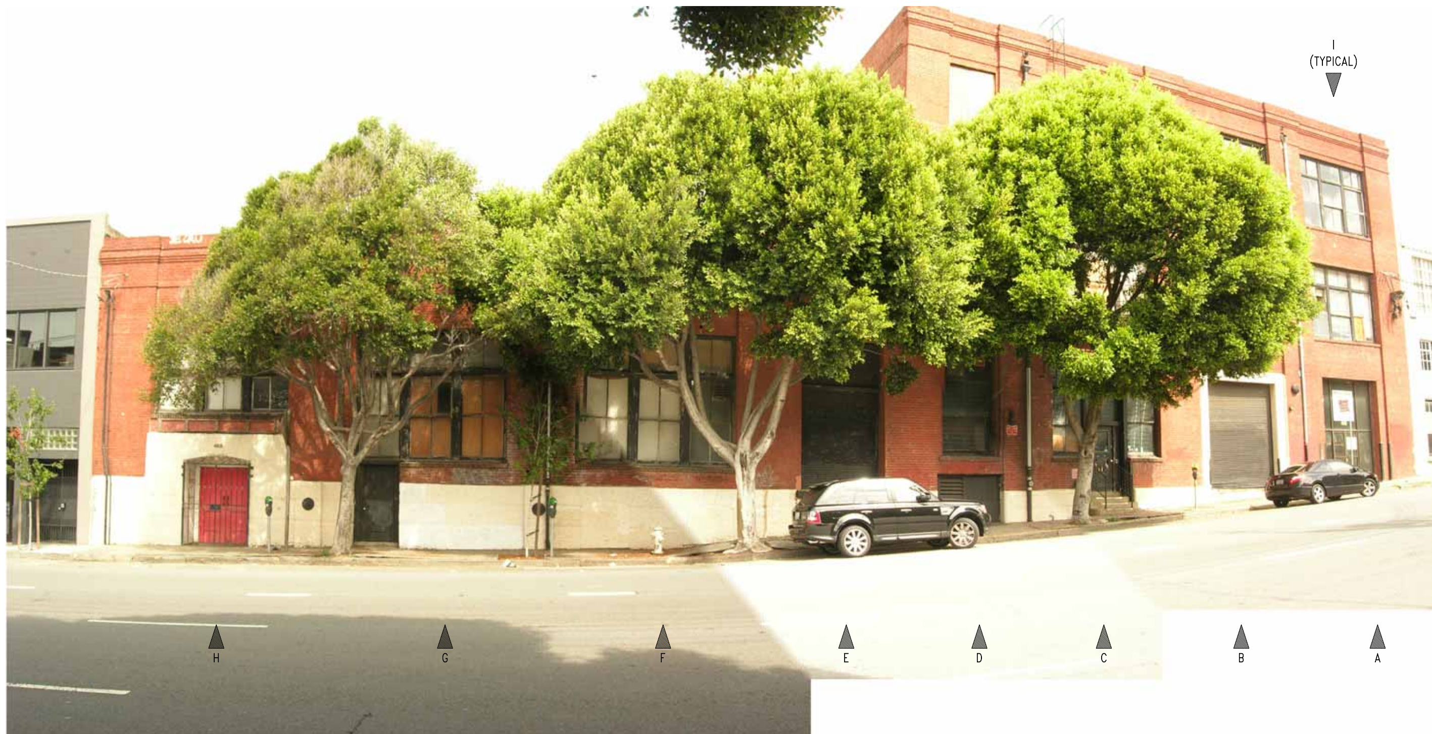
Bryant Street Elevation Panorama (View 04)
