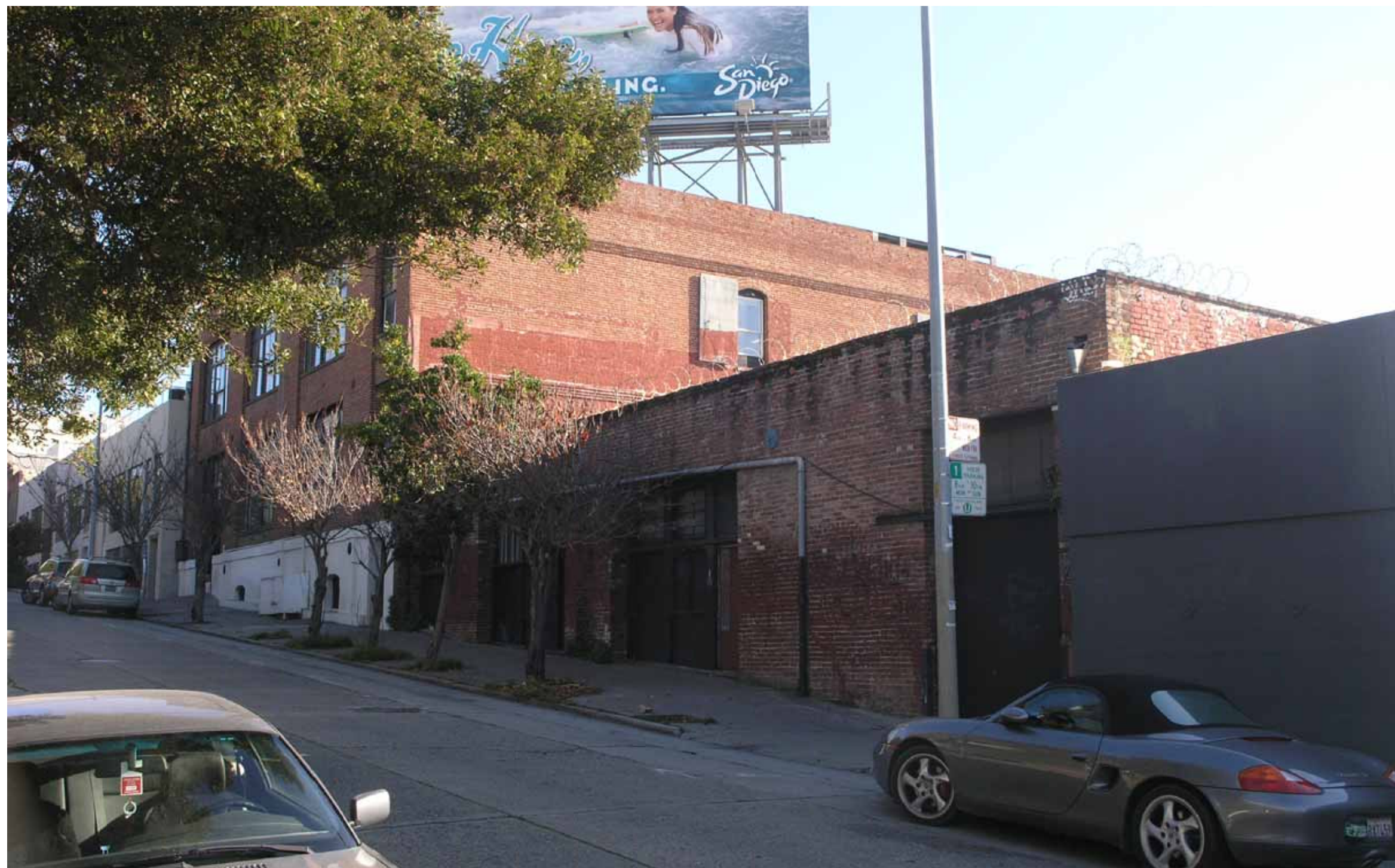
Stillman Streetwall & Context (View 05)
