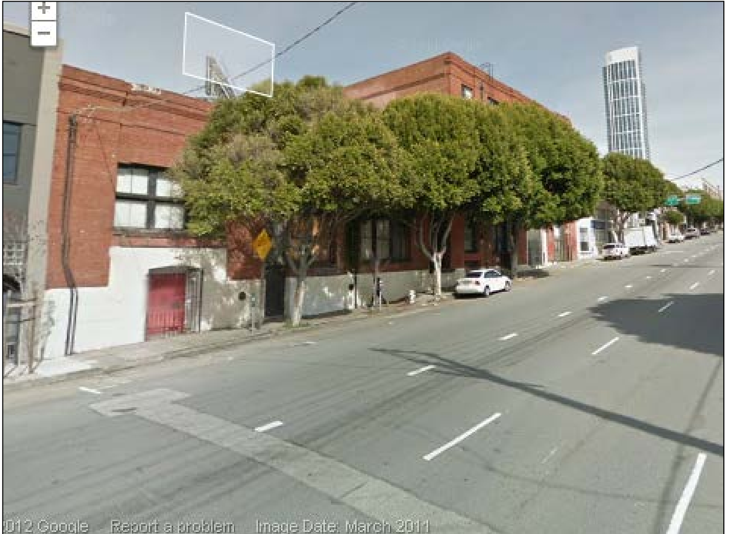
462 Bryant Street facade
