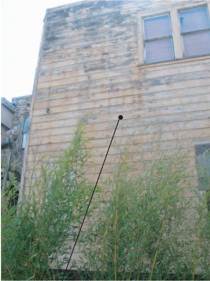
back of 711 Valencia (commercial building)
