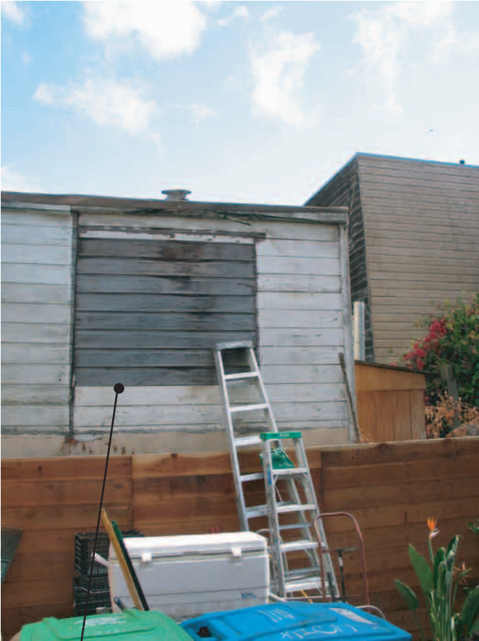
side of building at 116 Lexington Street 4
