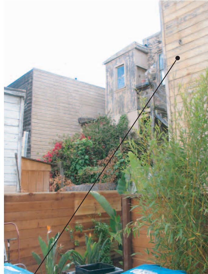
back of 711 Valencia (commercial building) 6
