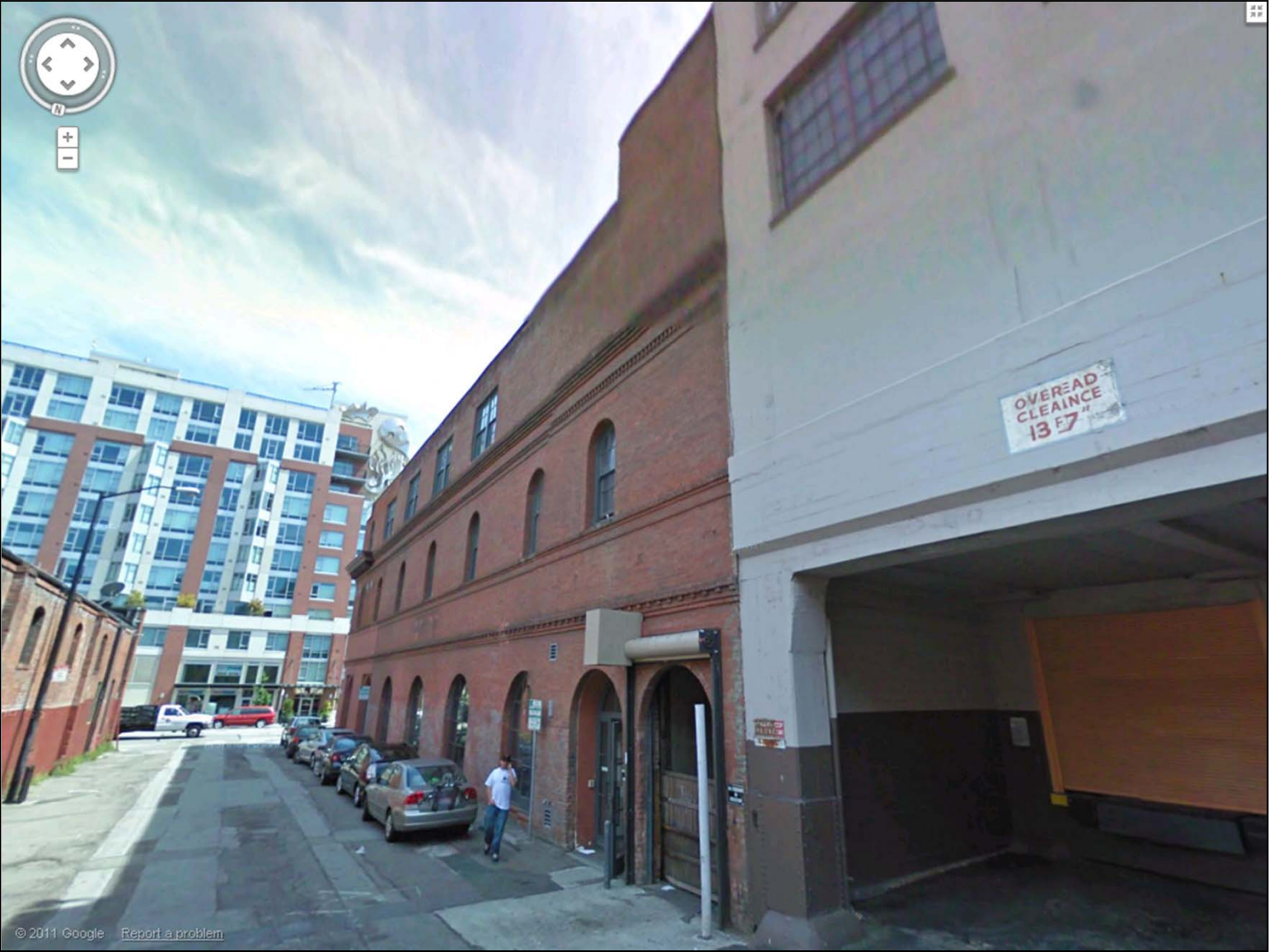
180 Townsend Street, View of Clarence Place Facade
