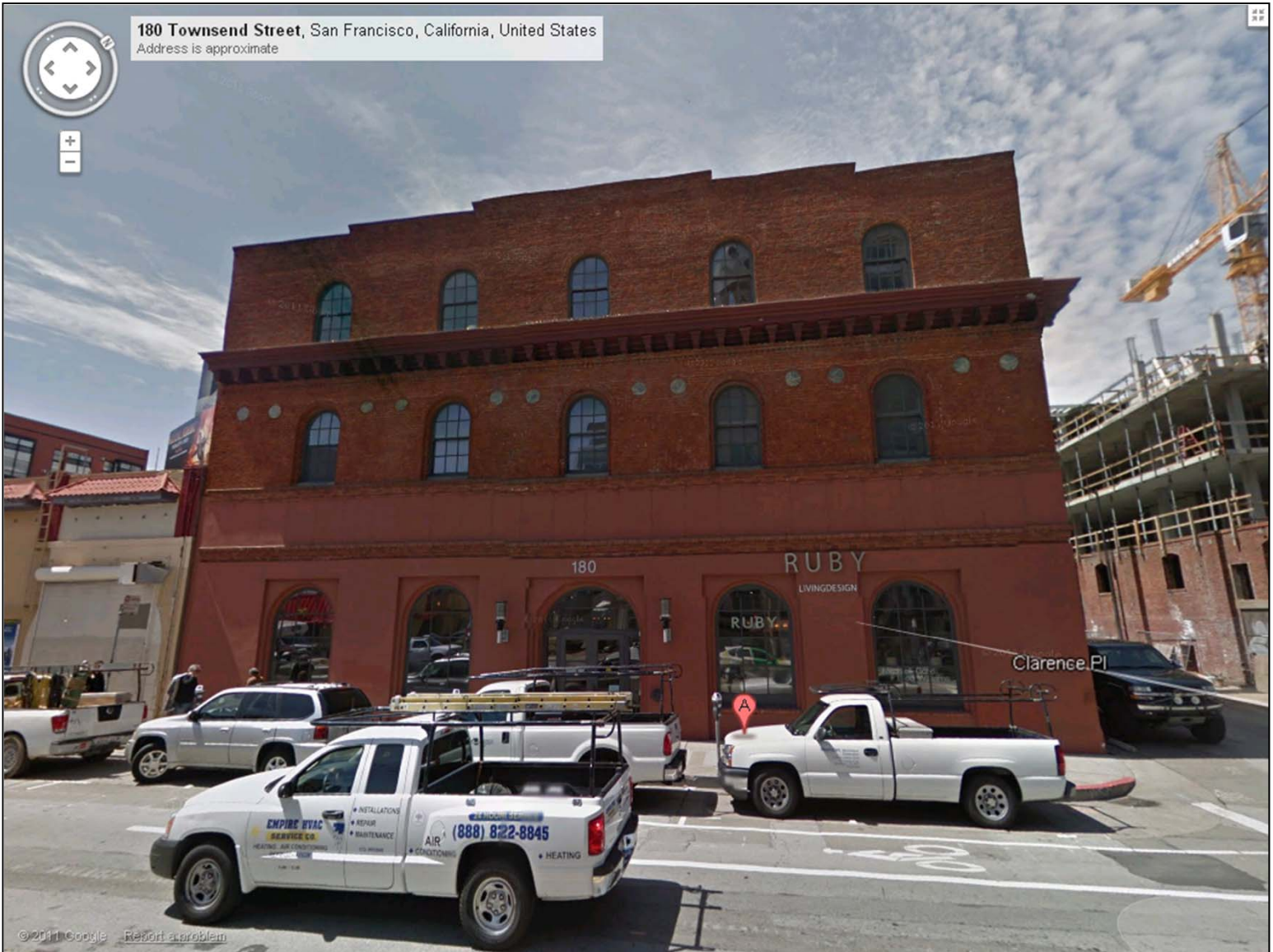
180 Townsend Street, View of Townsend Street Facade
