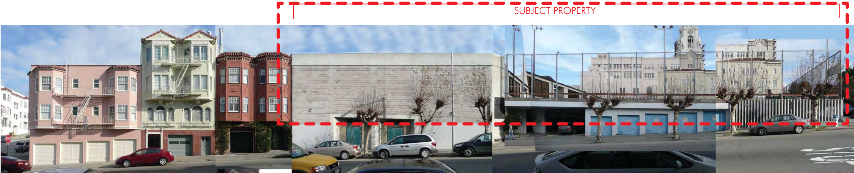
BLOCK PHOTO LOOKING EAST ON POWELL STREET
