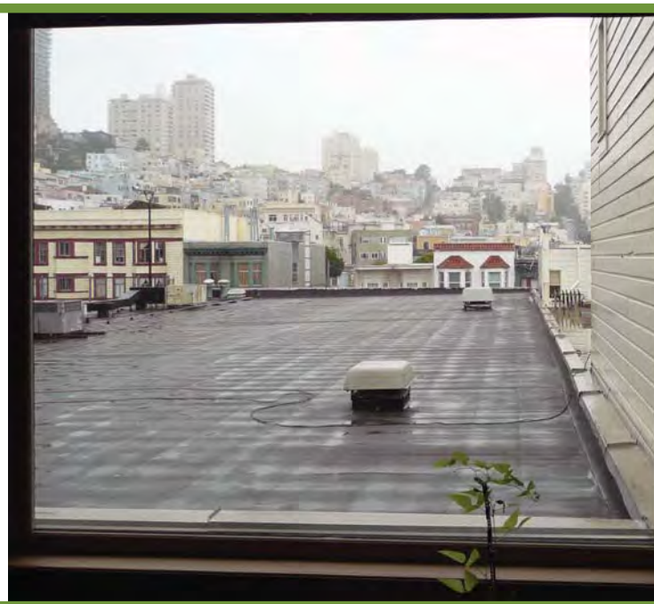
EXISTING VIEW LOOKING WEST
