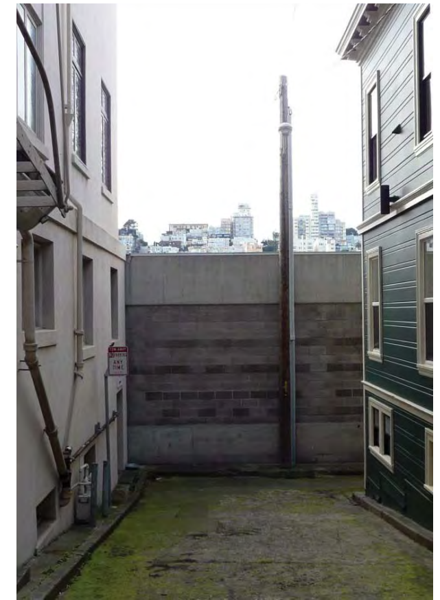
VIEW LOOKING AT NORTHEAST CORNER OF THE EXISTING STRUCTURE
