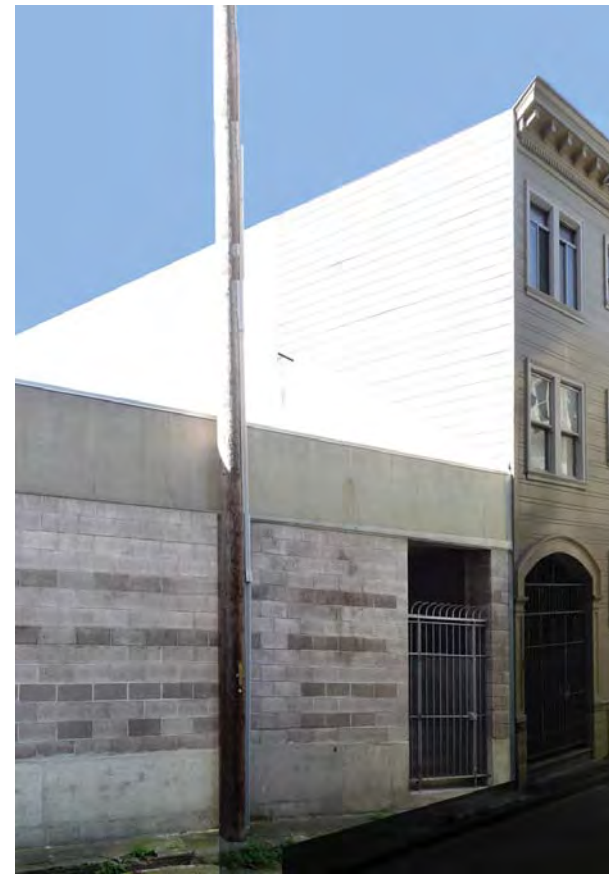
BLOCK PHOTO LOOKING WEST TOWARDS EAST SIDE OF THE PROPOSED STRUCTURE
