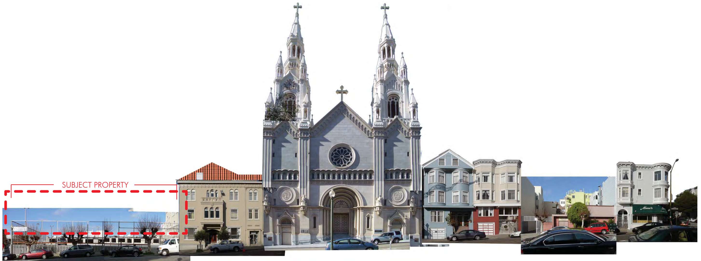
BLOCK PHOTO LOOKING EAST ON FILBERT STREET
