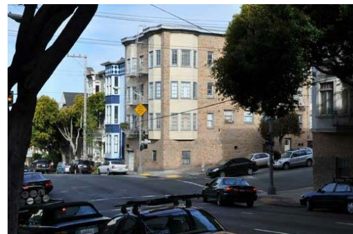
CORNER OF LAGUNA AND OAK STREET, SOUTHEAST CORNER
