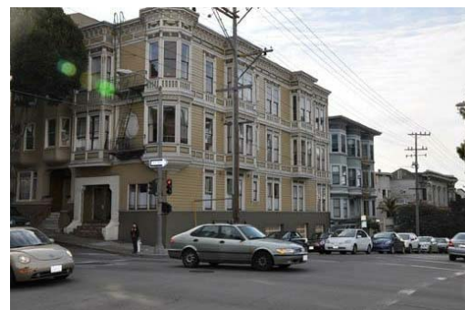
LAGUNA STREET AT OCTAVIA, NORTHWEST CORNER
