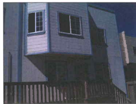
8 - NORTHEAST VIEW AT REAR
