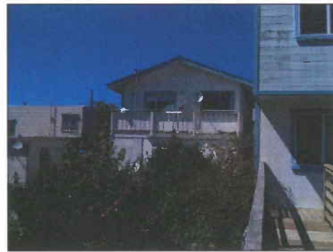
6 - NORTHWEST VIEW AT REAR
