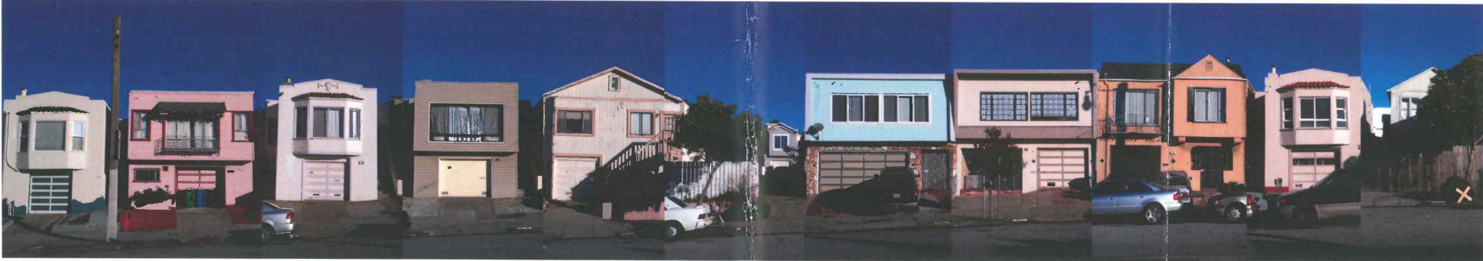
Cross Street View
