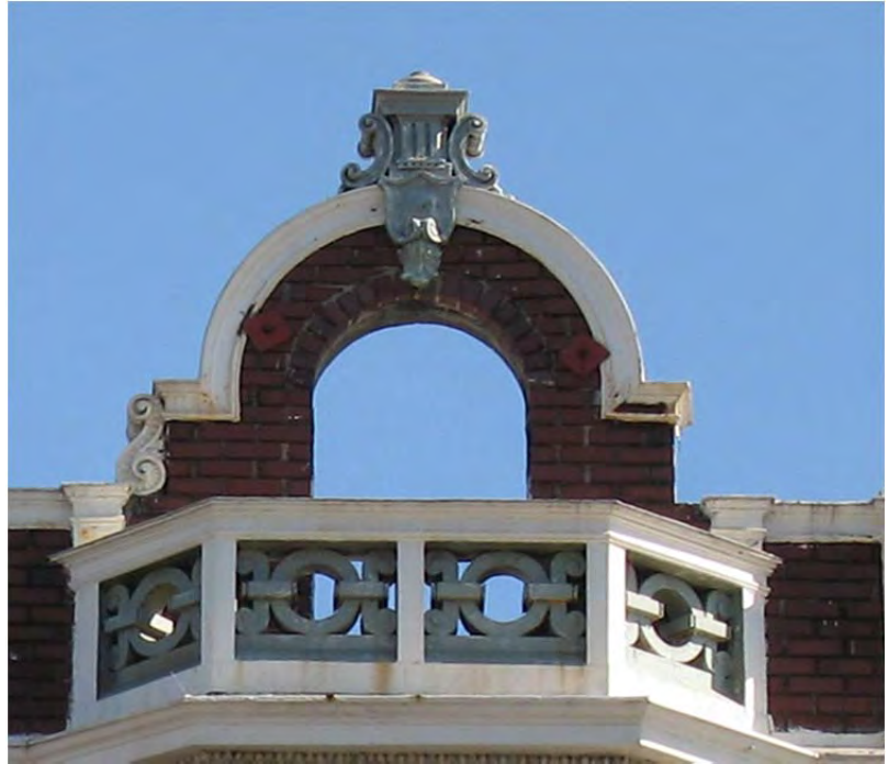
Figure 28 - 1693 Market St, parapet detail
