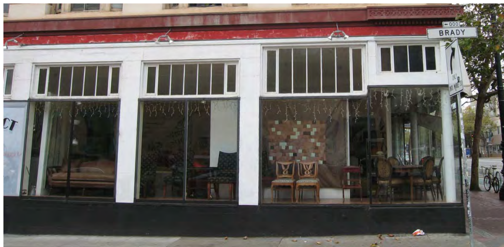
Figure 32 - 1649 Market Street, storefront detail
