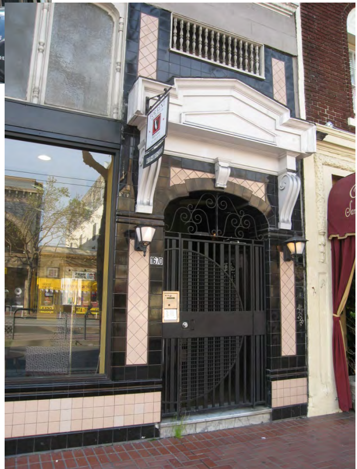
Figure 22 - 1670 Market Street entry detail
