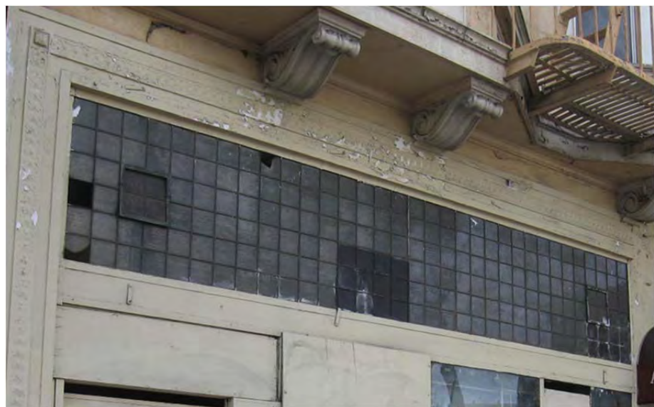
Figure 13 - 1657 Market Street storefront detail
