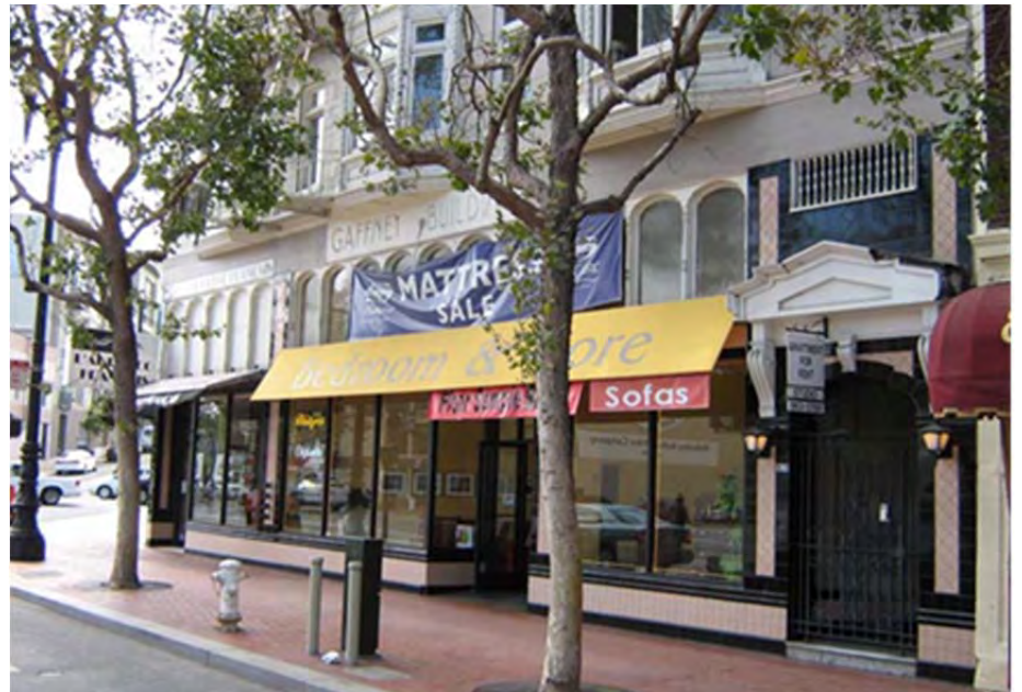
Figure 19 - 1670 Market Street, storefront detail
