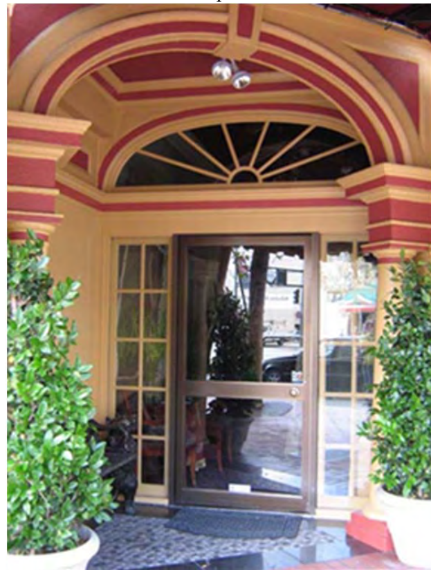
Figure 17 - 1666 Market Street, entry detail
