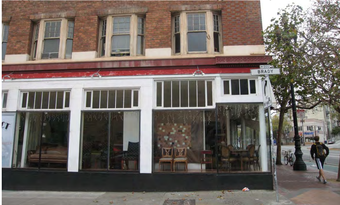
Figure 11 - 1649 Market Street, storefront detail
