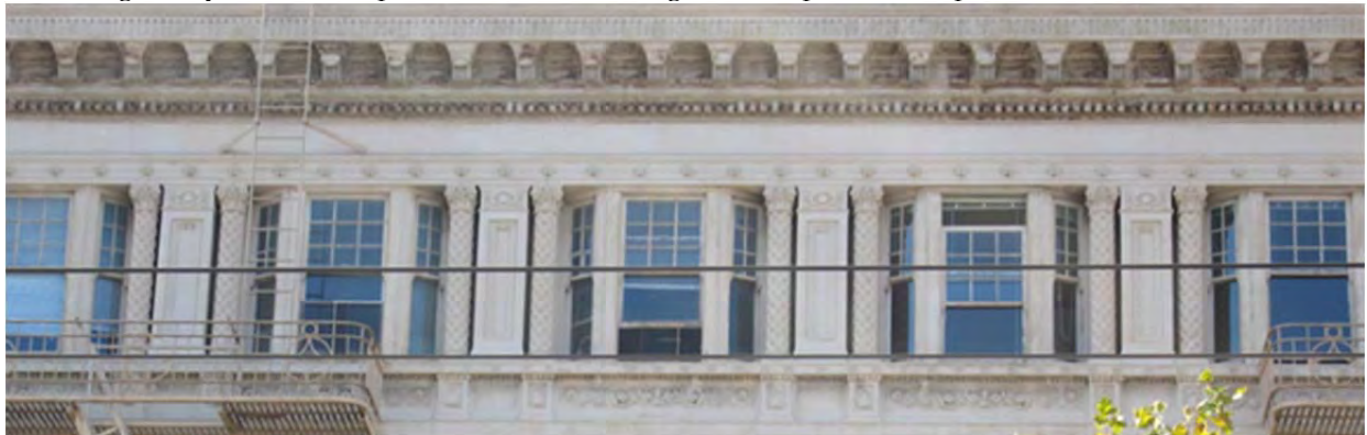
Figure 31 - 1649 Market Street, terra cotta 5th floor and metal entablature detail
