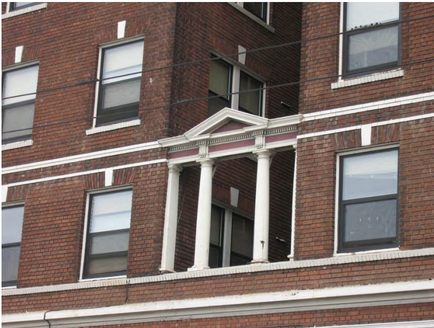
Figure 7 - 20 Franklin light court and pediment detail
