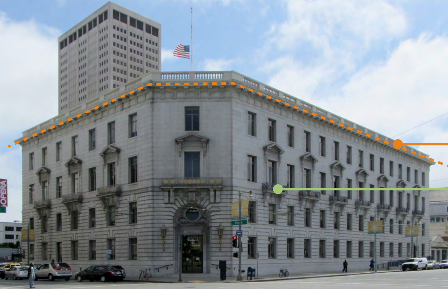
Cornice Line Continues Around the Building
