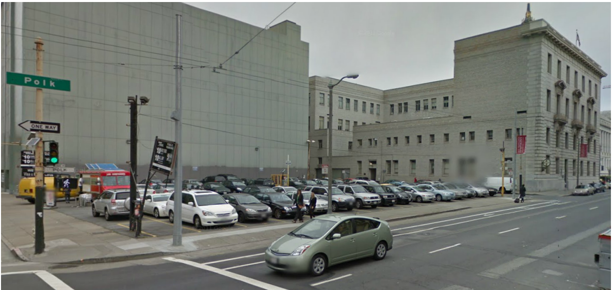
Figure 2b. View of existing surface parking lot at project site looking northwest
