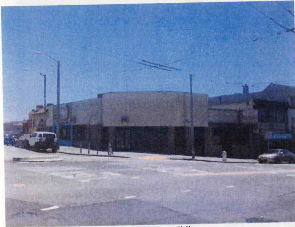
View of subject building
