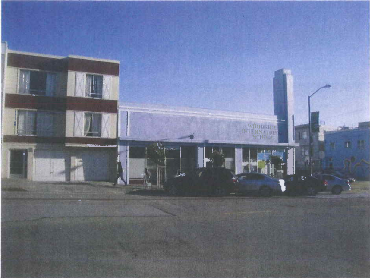
View of subject building
