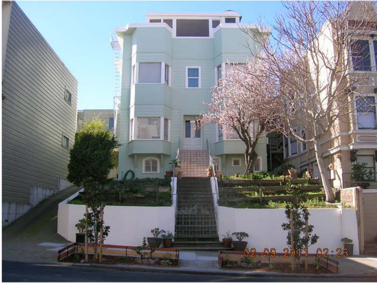
929 Broderick Street Front View
