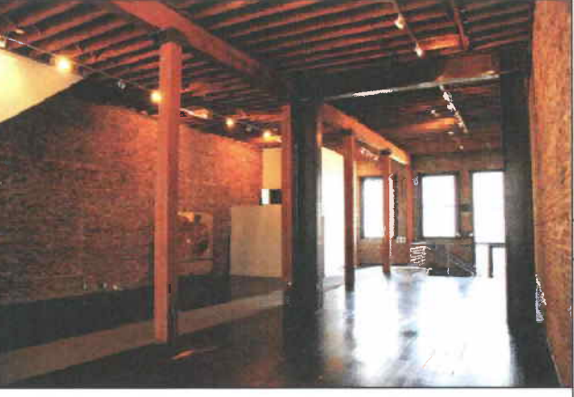
FIRST FLOOR INTERIOR - LOOKING SOUTH TOWARD MINNA STREET
