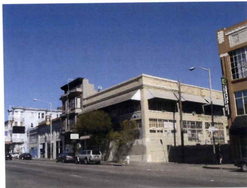
View from 9 th Street looking north east toward Clementina Street at easterly blockface
