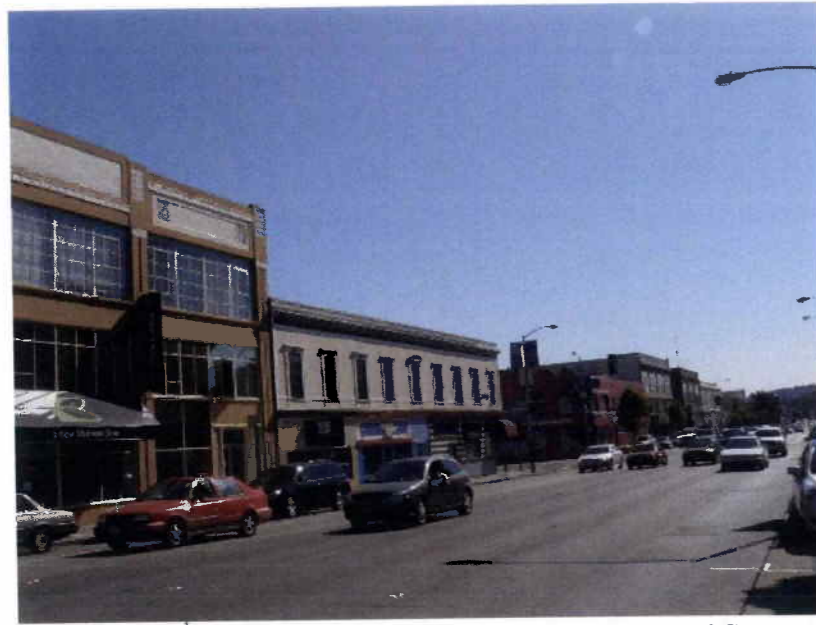
View from 9 th Street looking southeast toward Howard Street at easterly blockface
