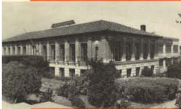
Administration building back of which is the manufacturing plant.
