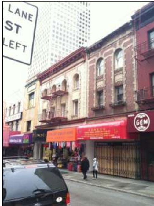
Neighboring buildings on Grant Street to the North
