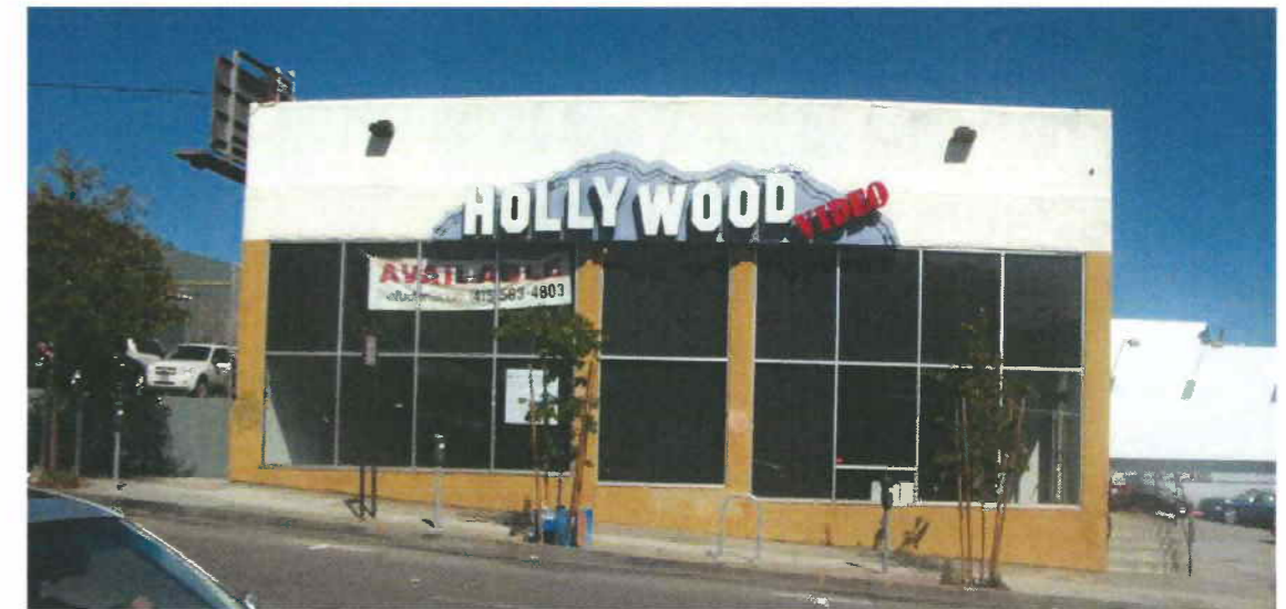
Subject property is on the south end of the block at the corner of South Van Ness Ave. and Cesar Chavez St.
