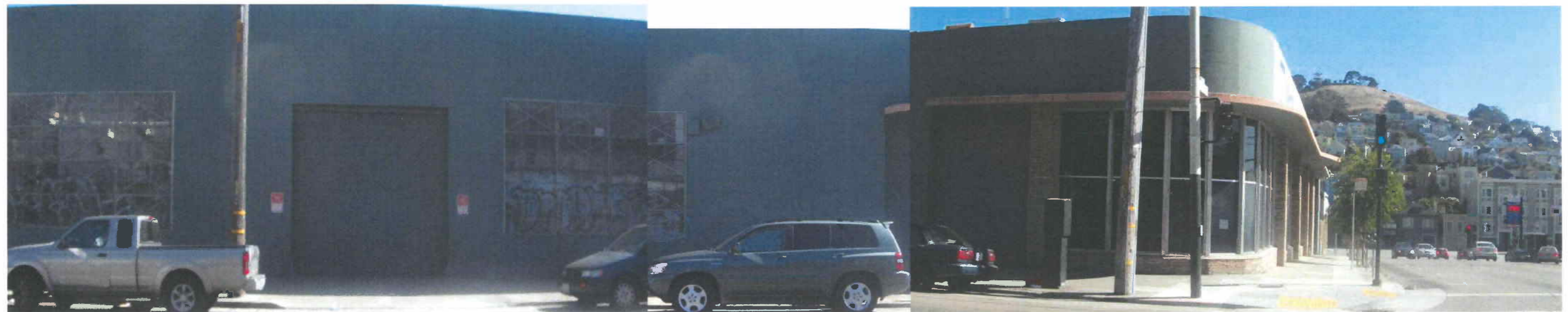
McMillan Electric shop entrance for contractor's vehicles and supplies. The right corner of the building contains offices for the contracting/engineering staff.
