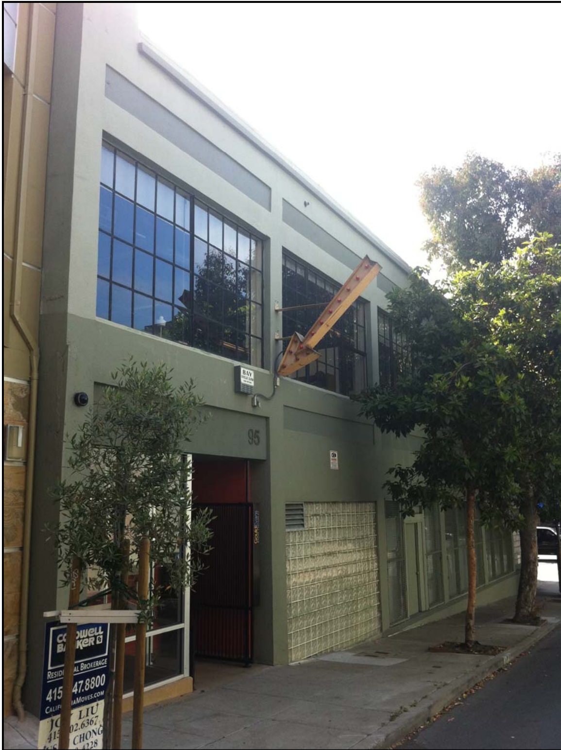
View of Subject Building along Brady Street
