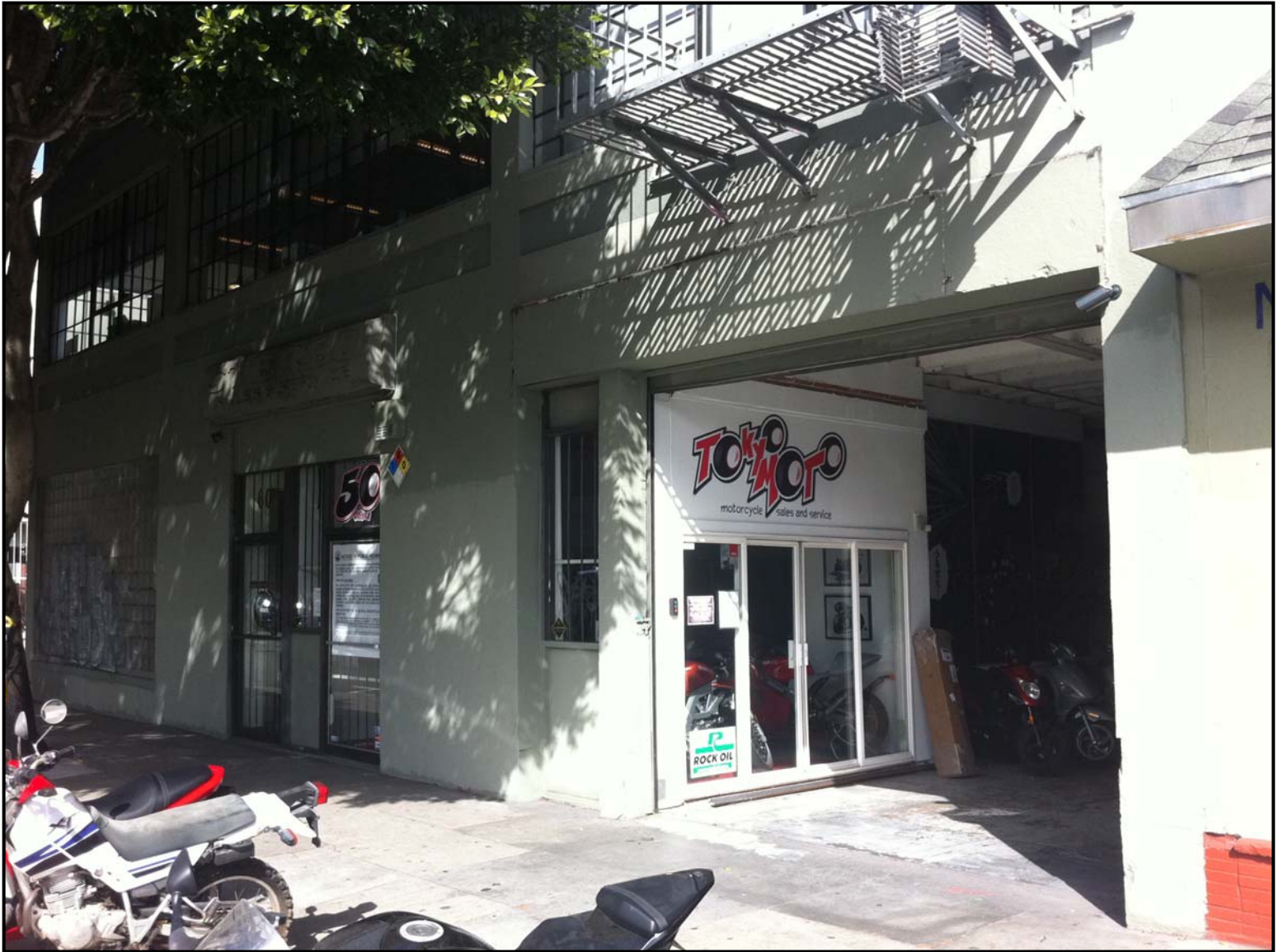
View of tenant space and storefront along Otis Street, 50 Otis Street
