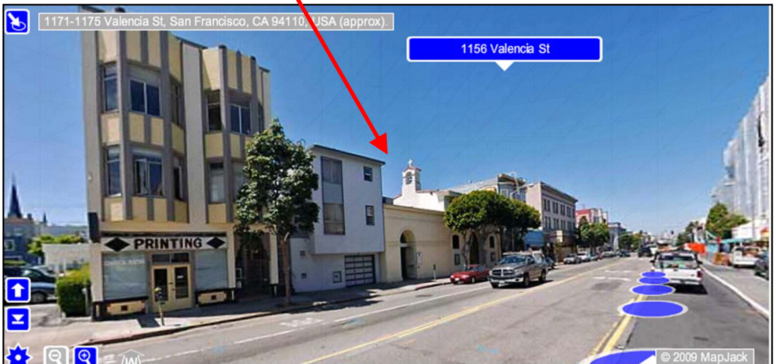
View of 1156 Valencia Street along Valencia Street
