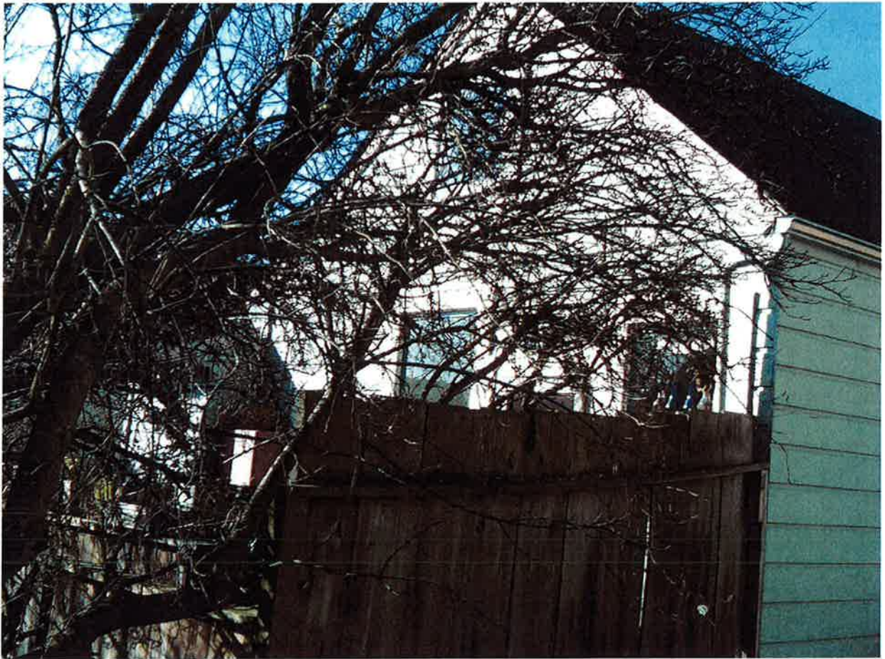
149 Andover St, Rear, adjacent to the south
