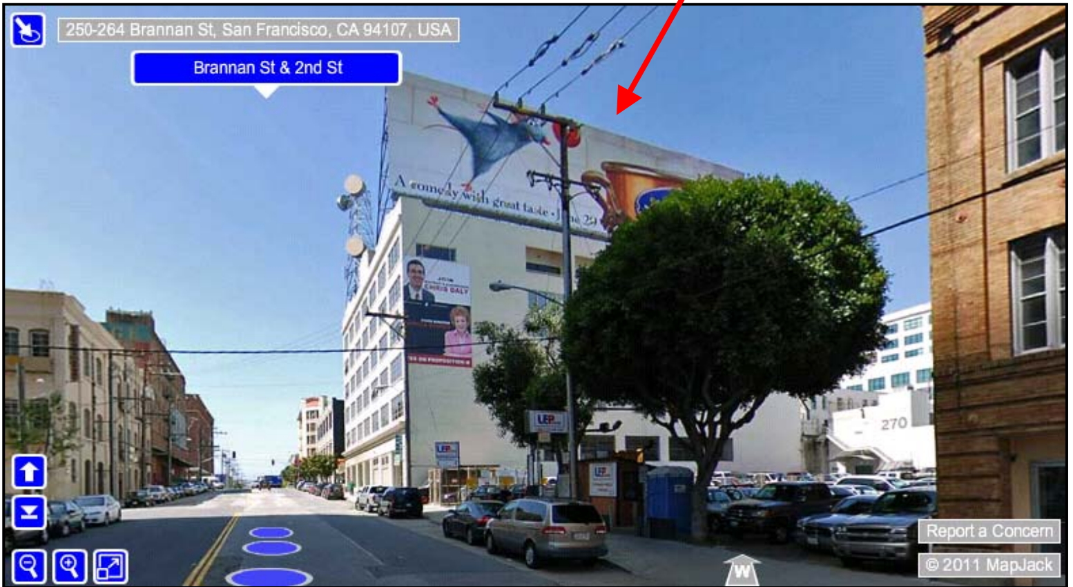
View looking west along Brannan Street showing 274 Brannan and existing billboard and antenna tower
