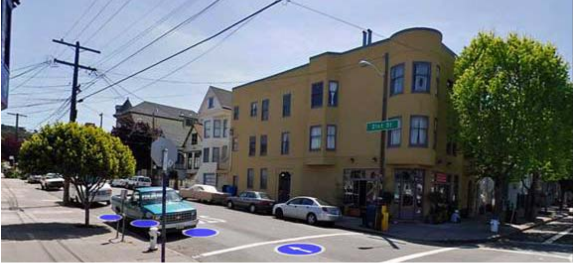
Properties to the Southeast Corner
