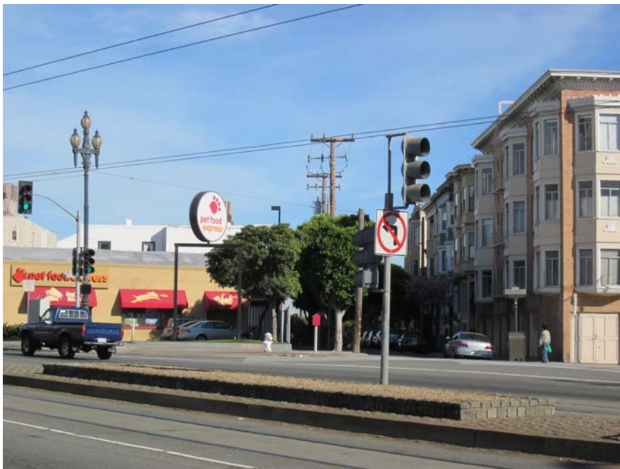
View toward Subject building across Market, East down Clinton Park
