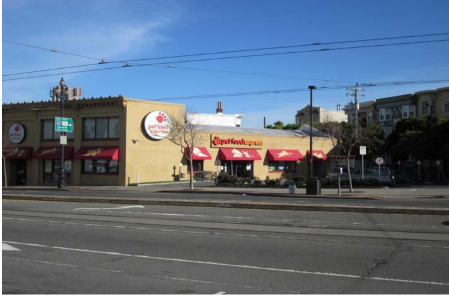
View toward adjacent building (existing antennas in background) SE across Market
