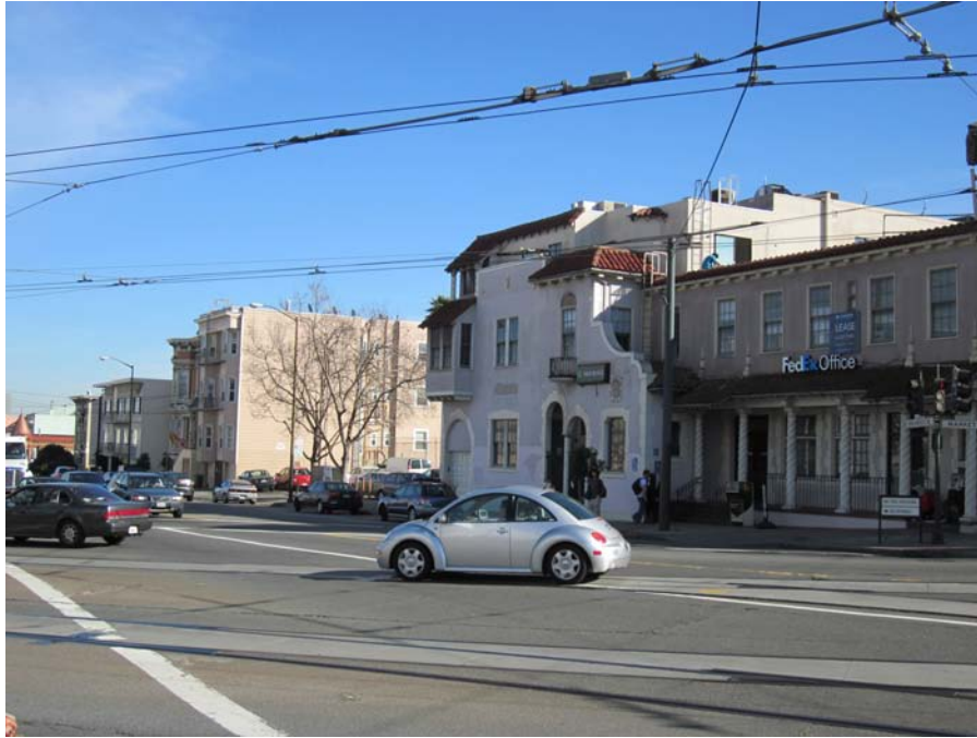
View of Subject building looking East on Duboce
