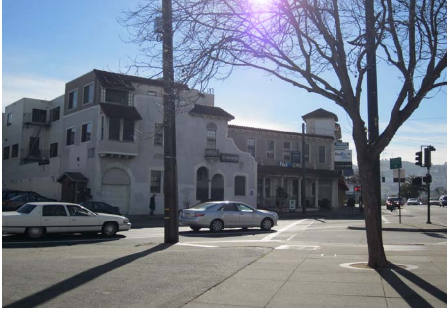
View West toward subject building from corner of Market and Duboce
