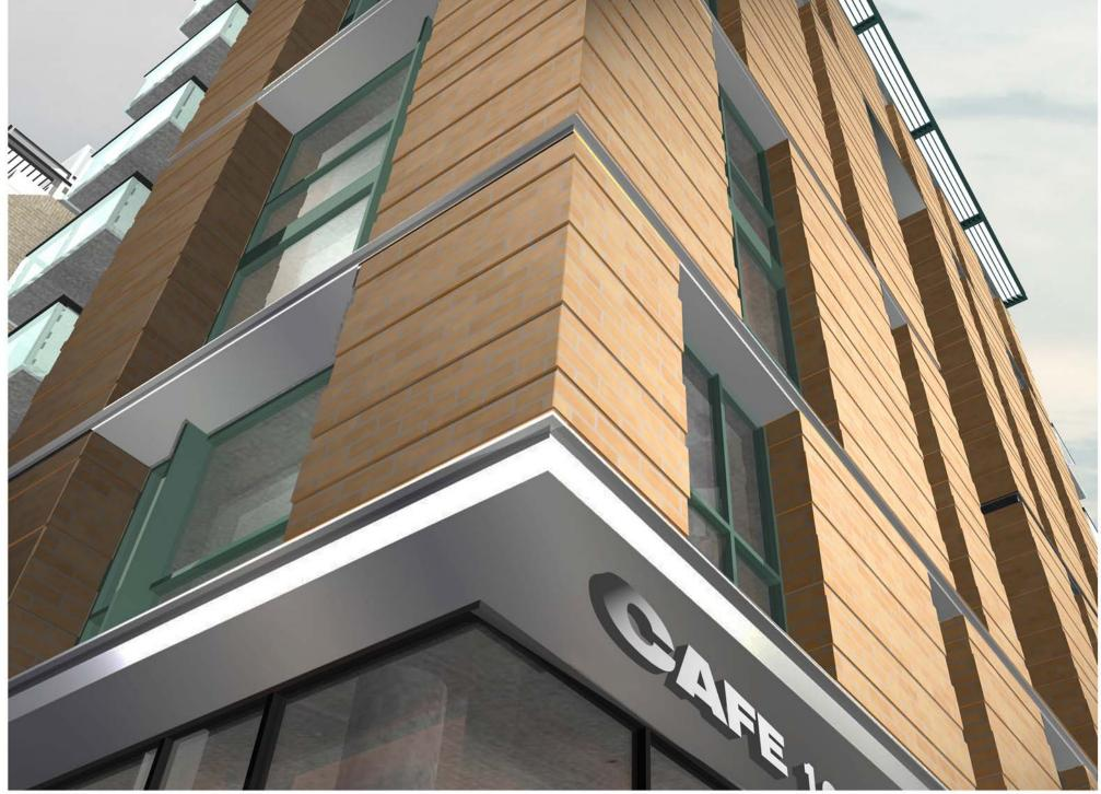
Detail View brick cladding w/ alternating thickess to create shadow and texture
