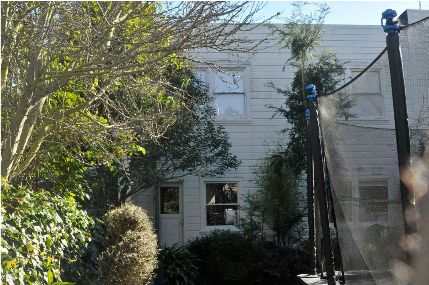
422 DAY STREET Rear Facade
