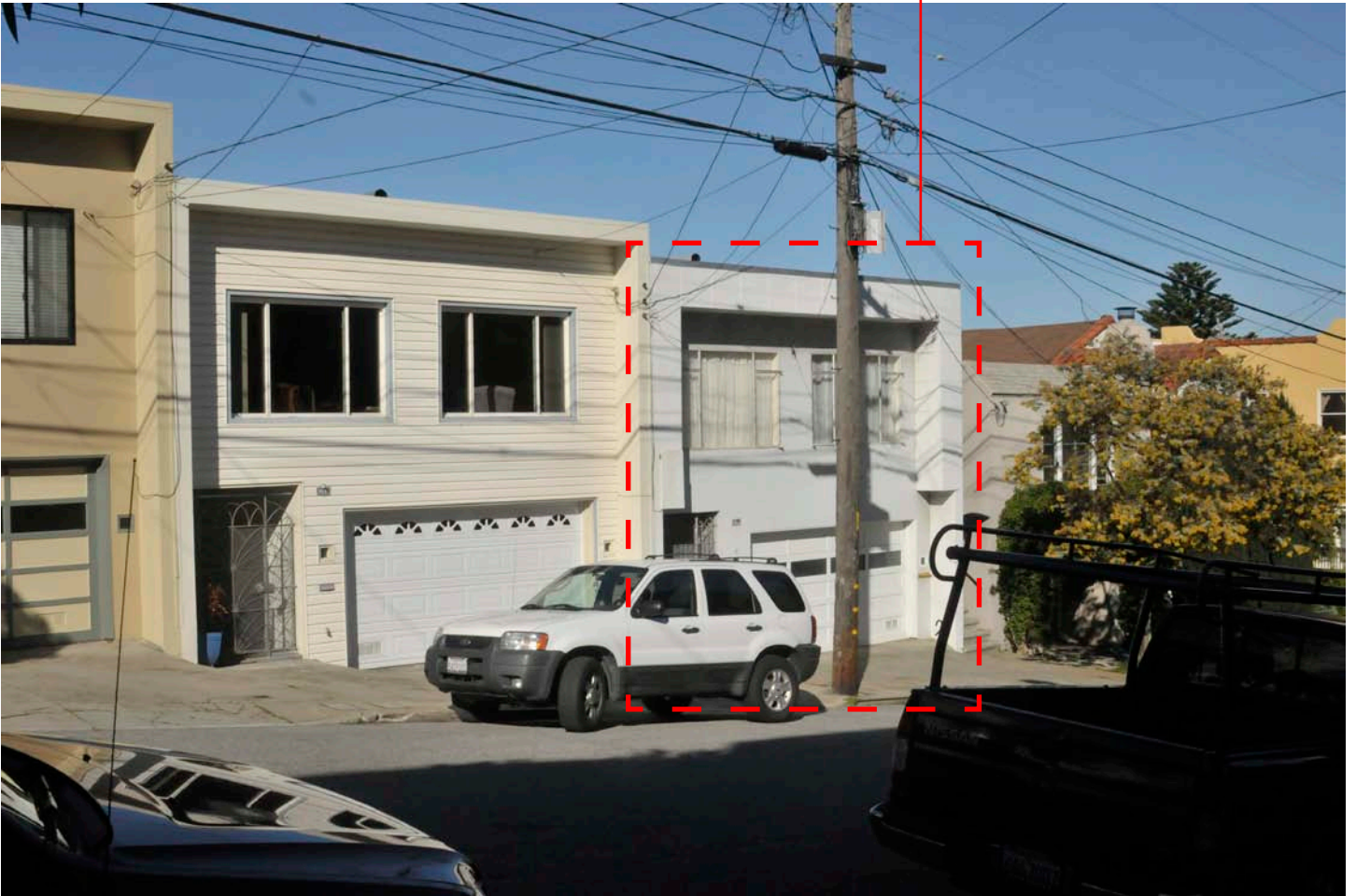
422 DAY STREET Front Facade
