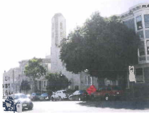
View of the western blockface of Larkin Street looking south from Vallejo Street
