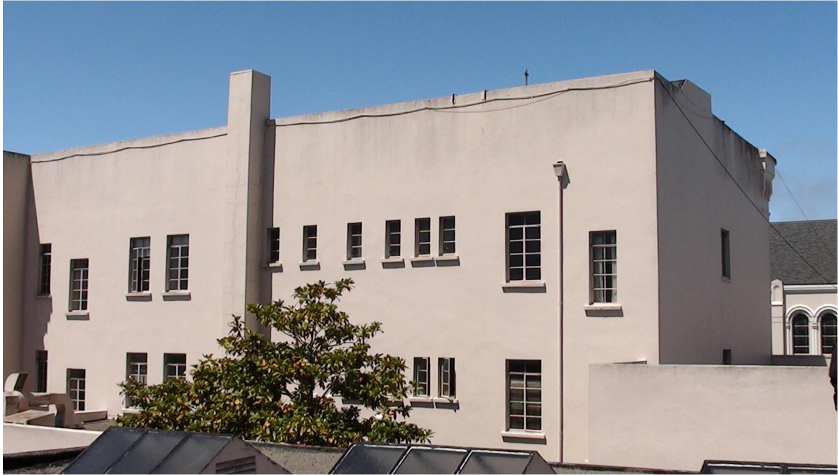
EXISTING CONDITIONS - WEST
