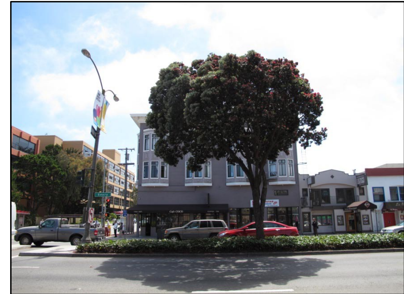
6TH AVE. & 4201 GEARY BLVD
