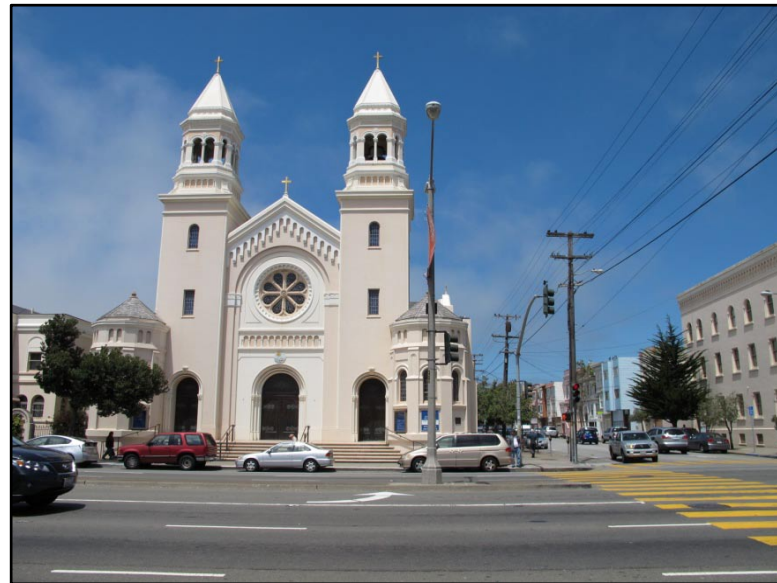
8TH AVE. & 4410 GEARY BLVD
