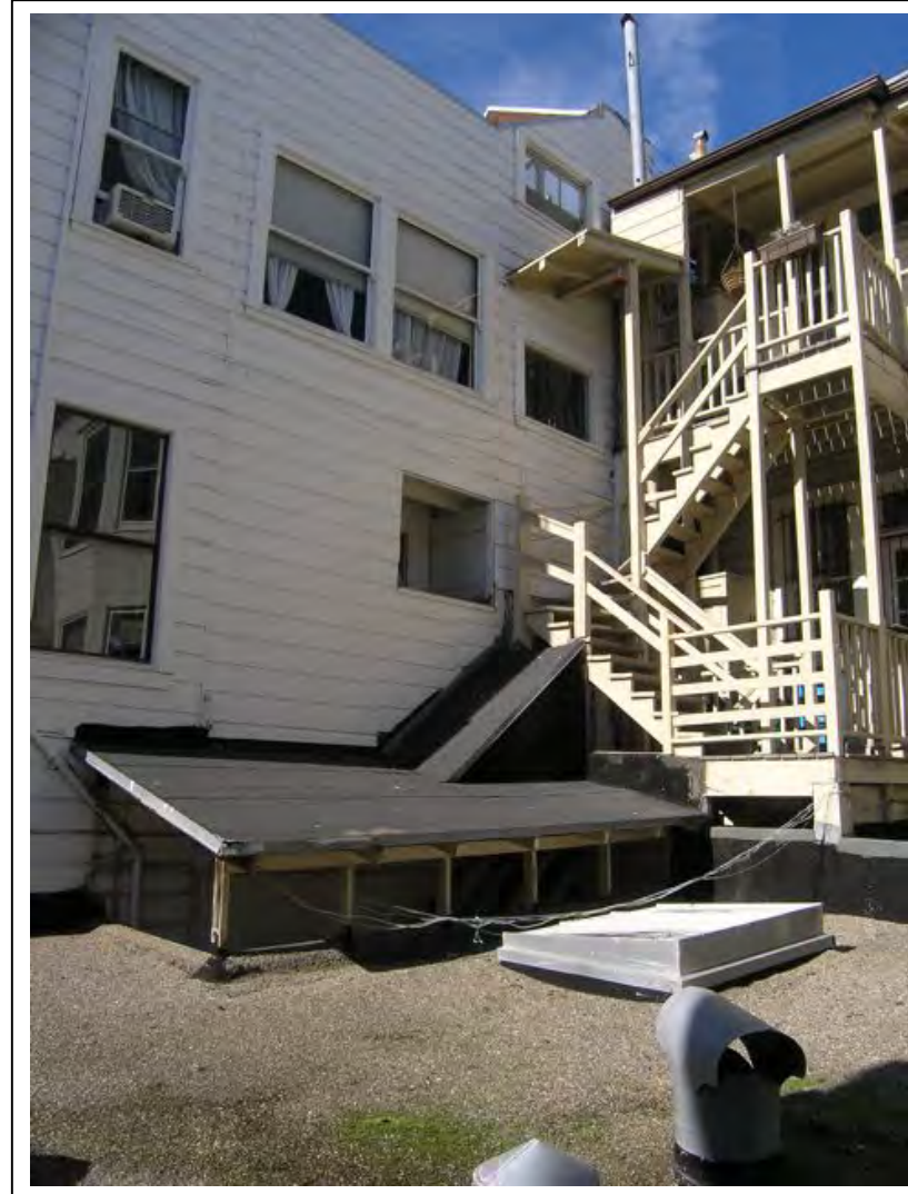
REAR VIEW LOOKING NORTHWEST.
