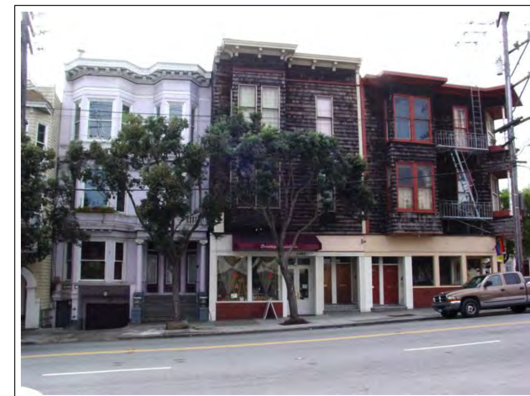
STREET VIEW OF 3489 16TH STREET.
