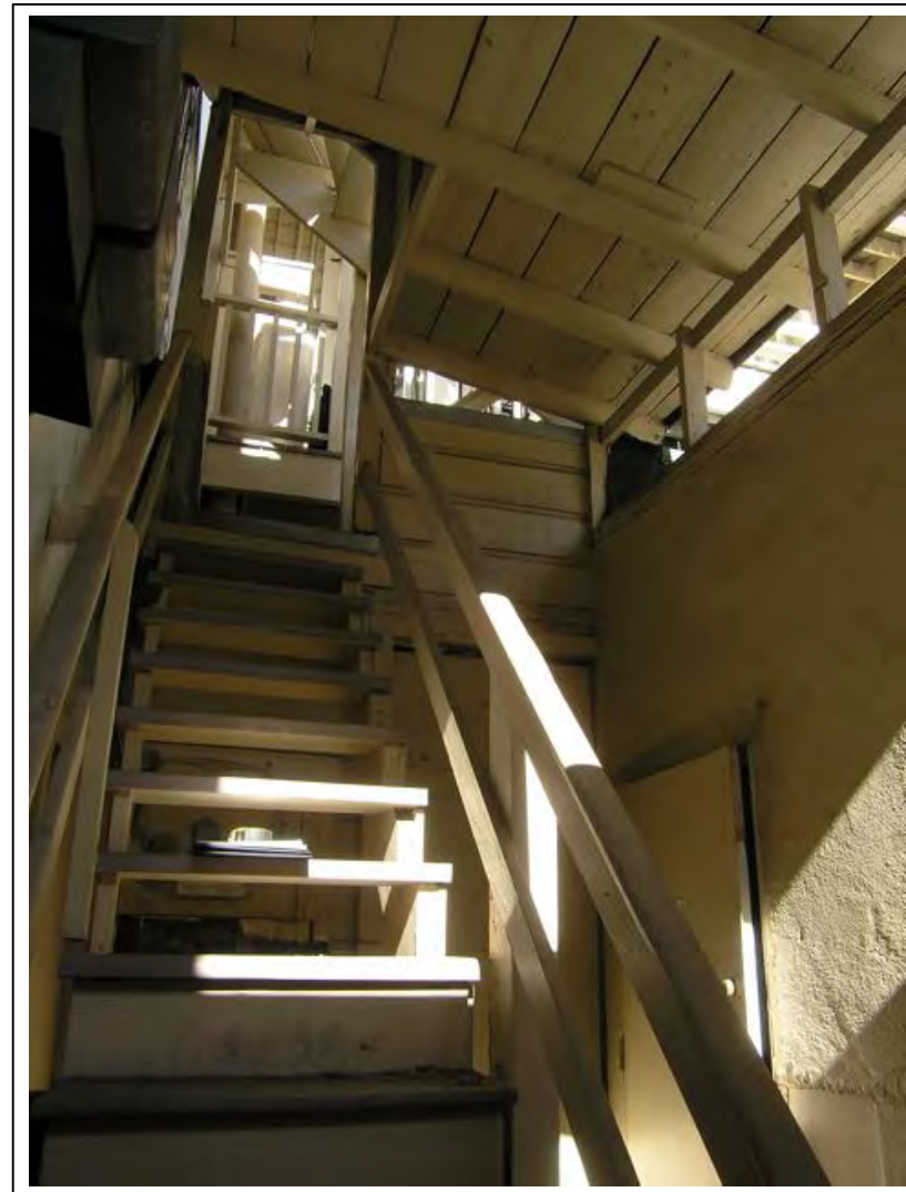
VIEW FROM EGRESS STAIR TO ROOF LEVEL.
