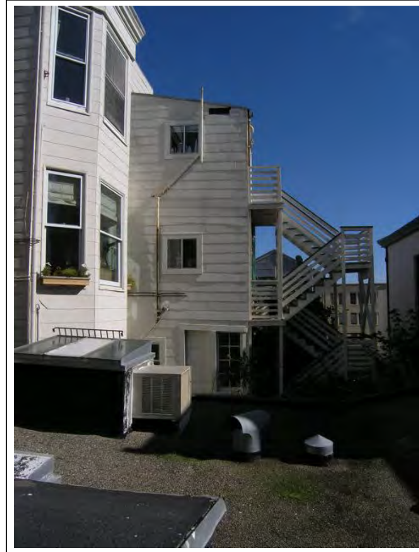
SIDE VIEW LOOKING EAST.
