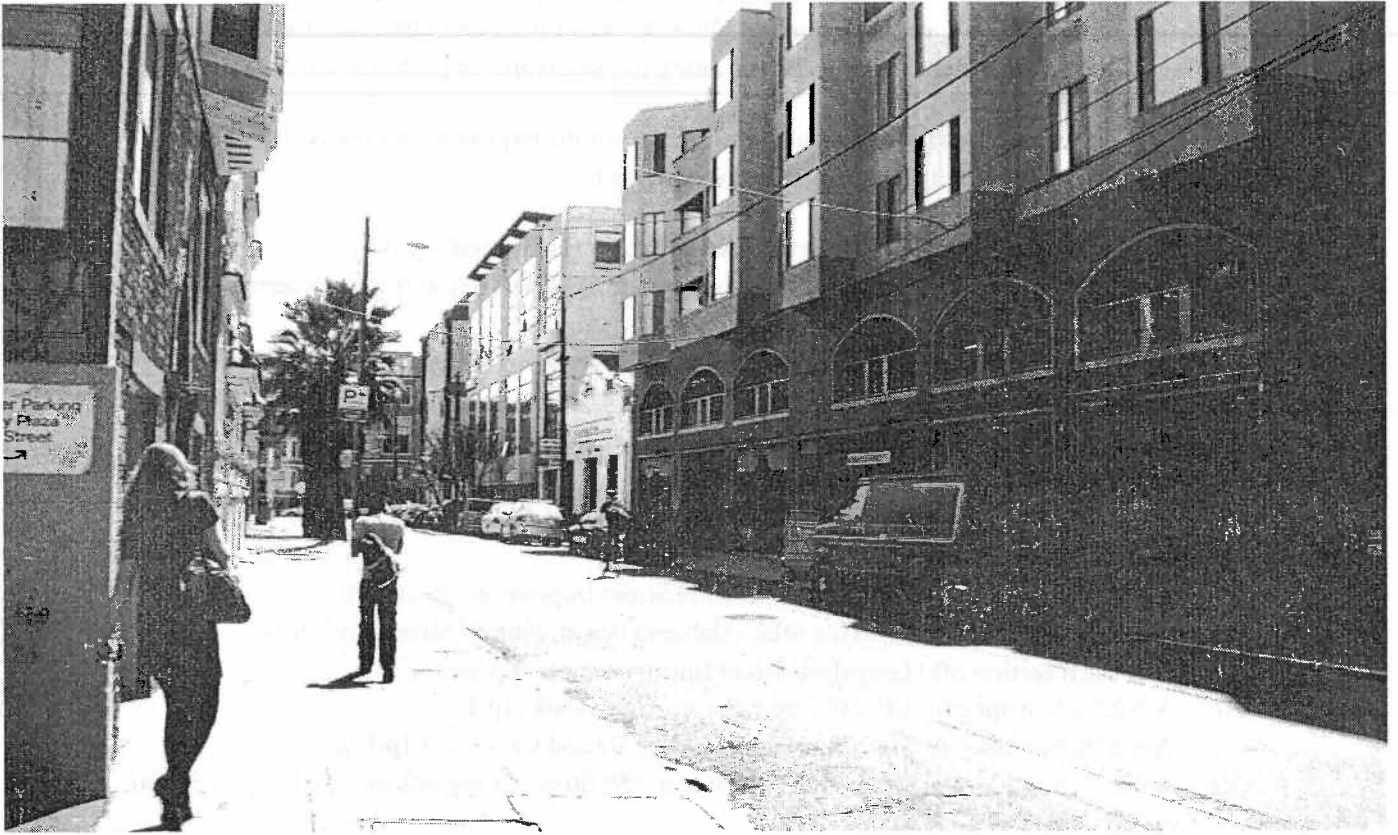
Figure E-2.2a: Existing Site-Specific Streetscape Improvement Project at Hoff and 16th Streets- Looking South.
