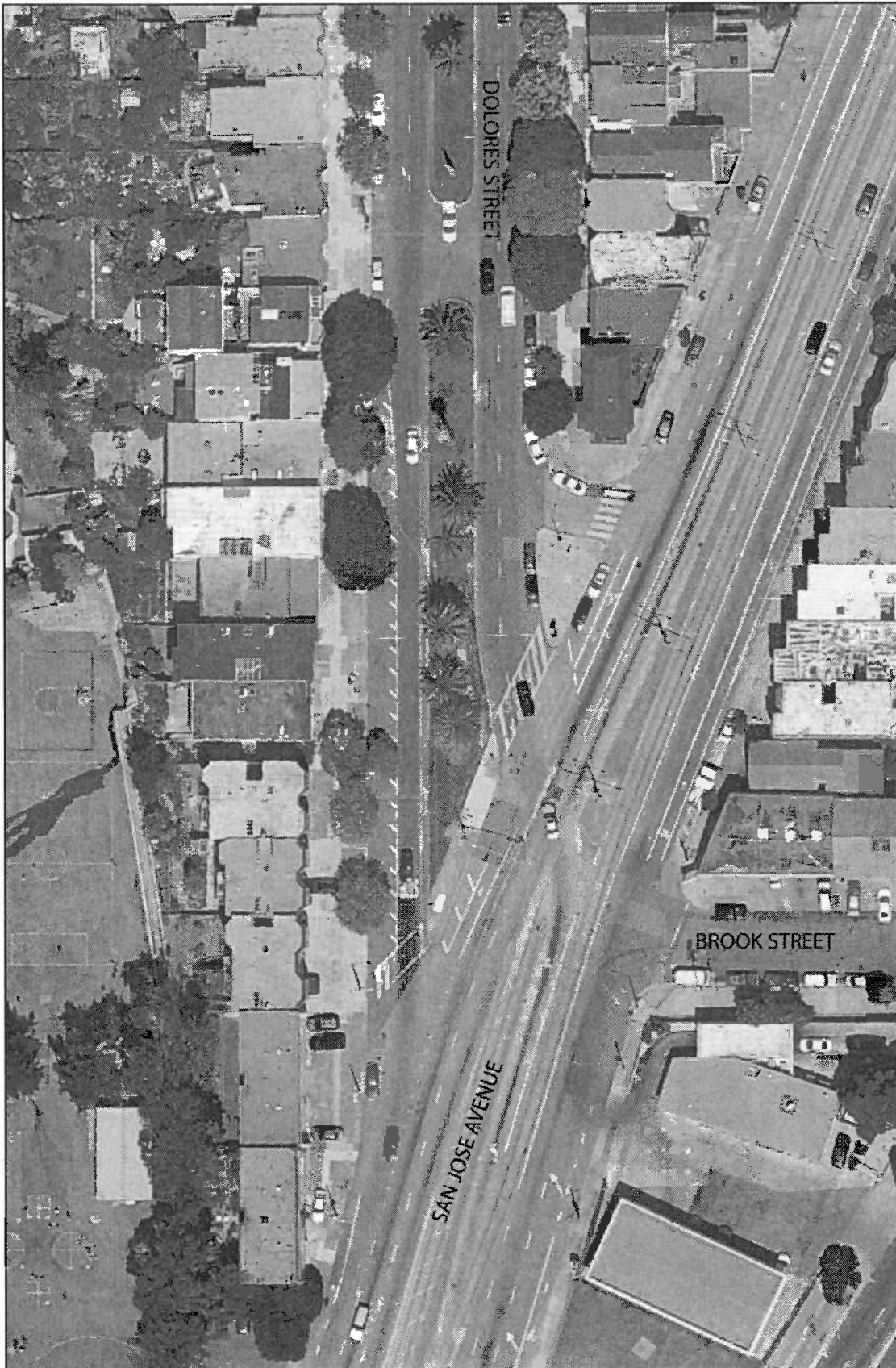
Figure 8: Dolores/ San Jose Intersection Existing Conditions
