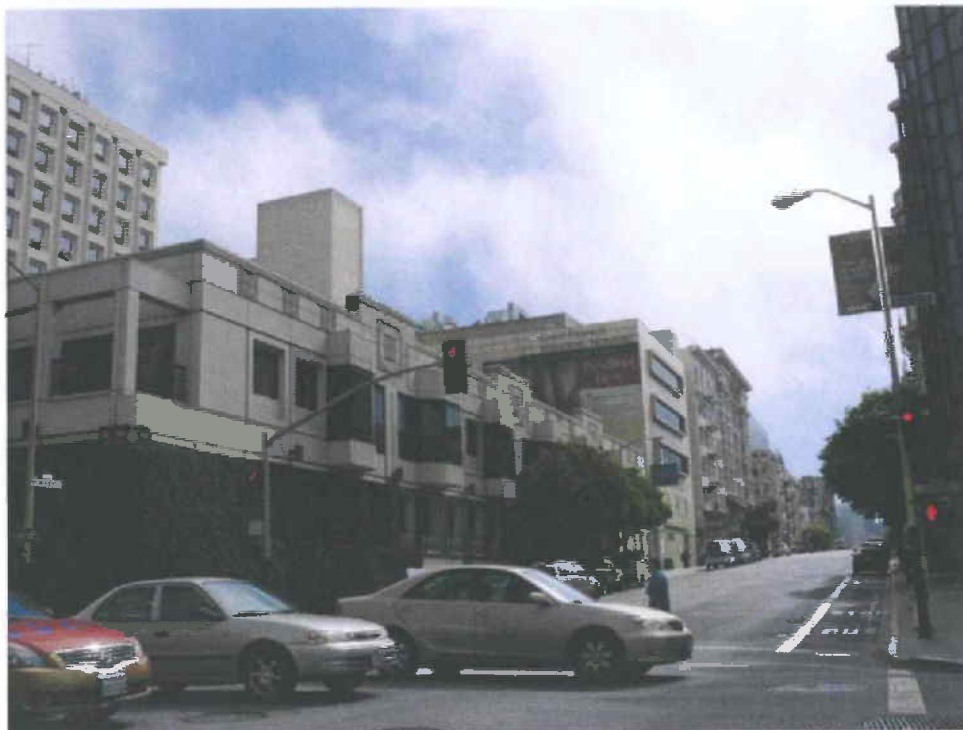
Looking east on Bush at northerly blockface from subject building
