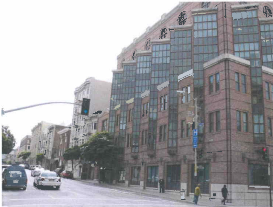
Looking east on Bush at southerly blockface
