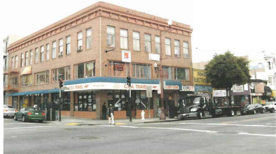
North-West View of Mission Street
