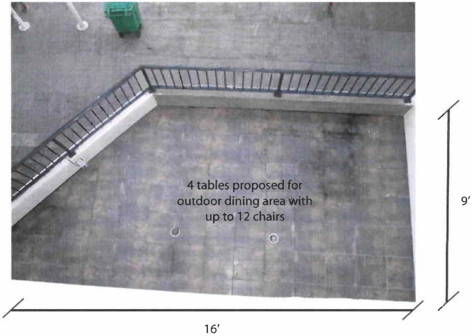
1787 Union Street Patio from roof
