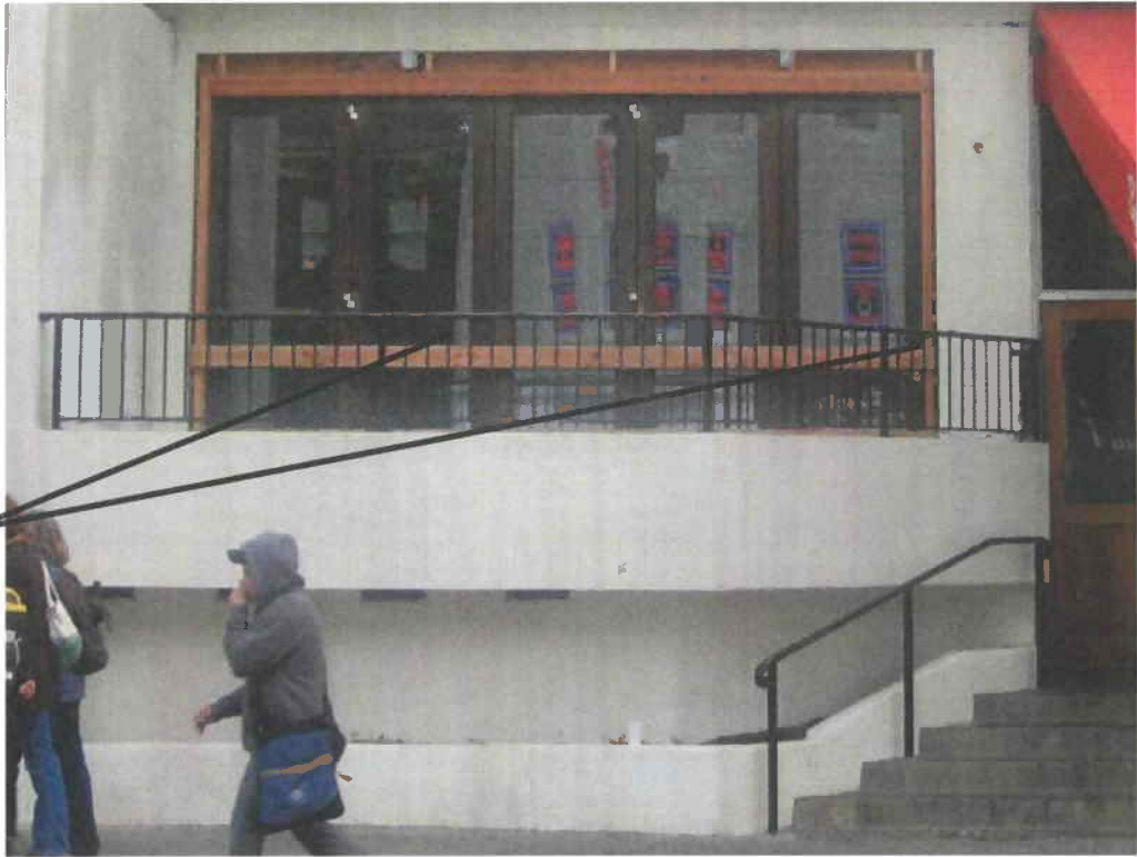
1787 Union Street Patio from street
