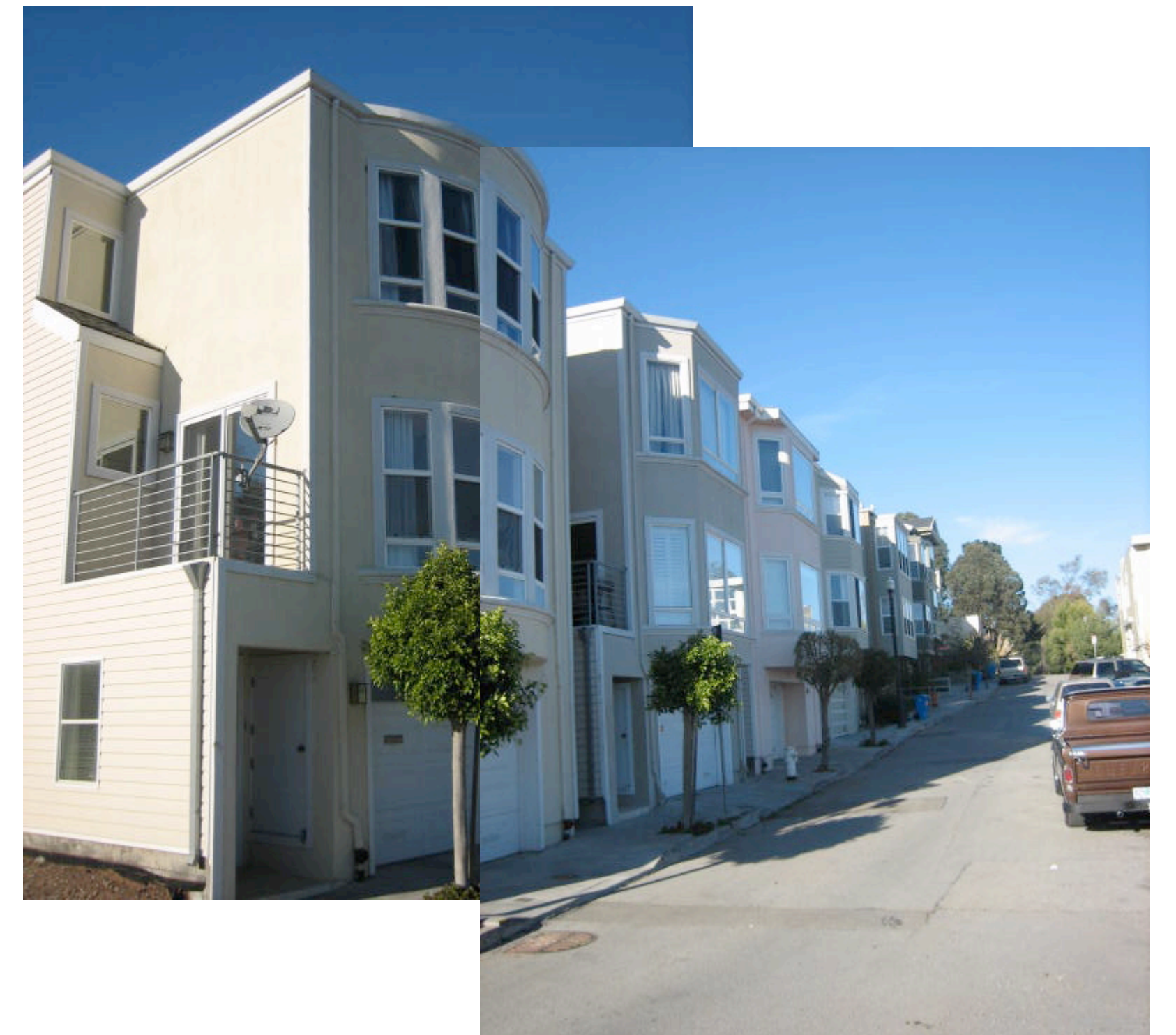
VIEW WEST/ NORTH (UP BREWSTER)
