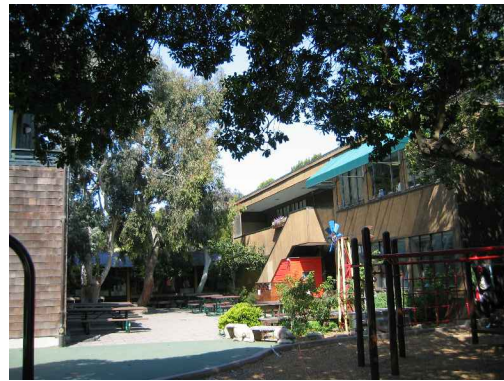
EXISTING HERBST BUILDING 7
