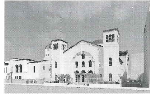
VIEW FROM VALENCIA STREET
