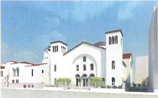
VIEW FROM VALENCIA STREET
