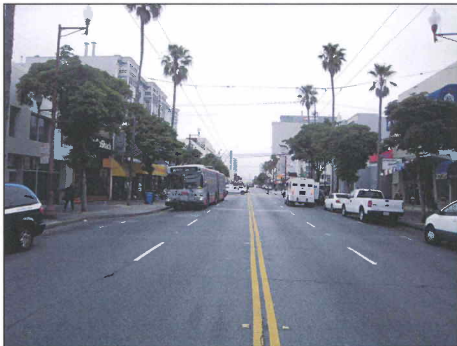
(C) FACING NORTH UP MISSION STREET
