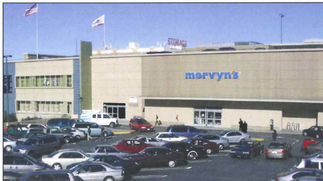
View of Existing Conditions Looking Northwest Toward Building at Parking Lot B.
