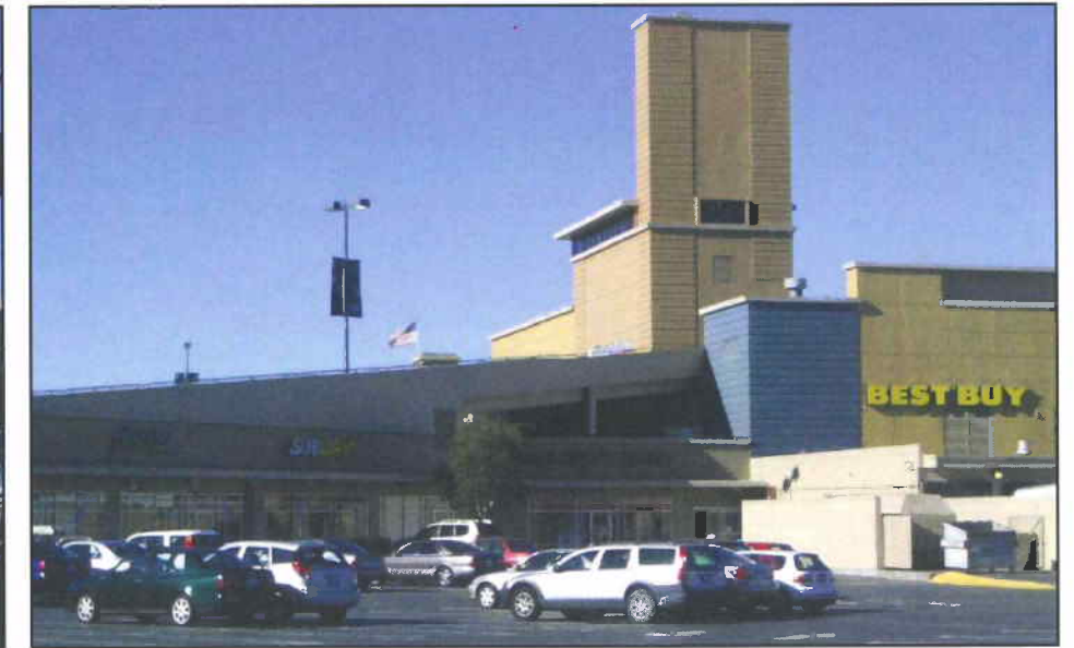
View of Existing Conditions Looking West Toward Building at Parking Lot E.
