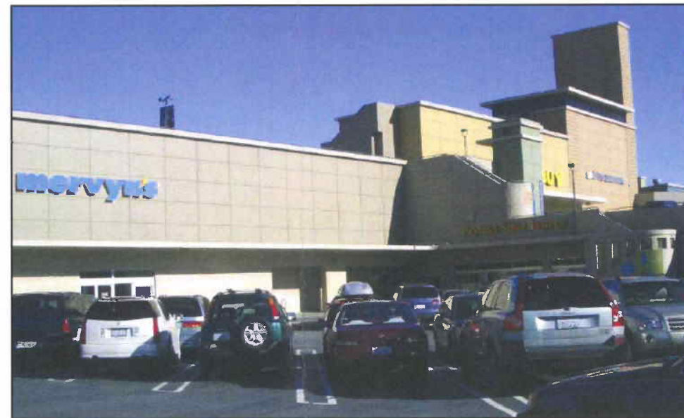
View of Existing Conditions Looking Northeast Toward Building at Parking Lot B.
