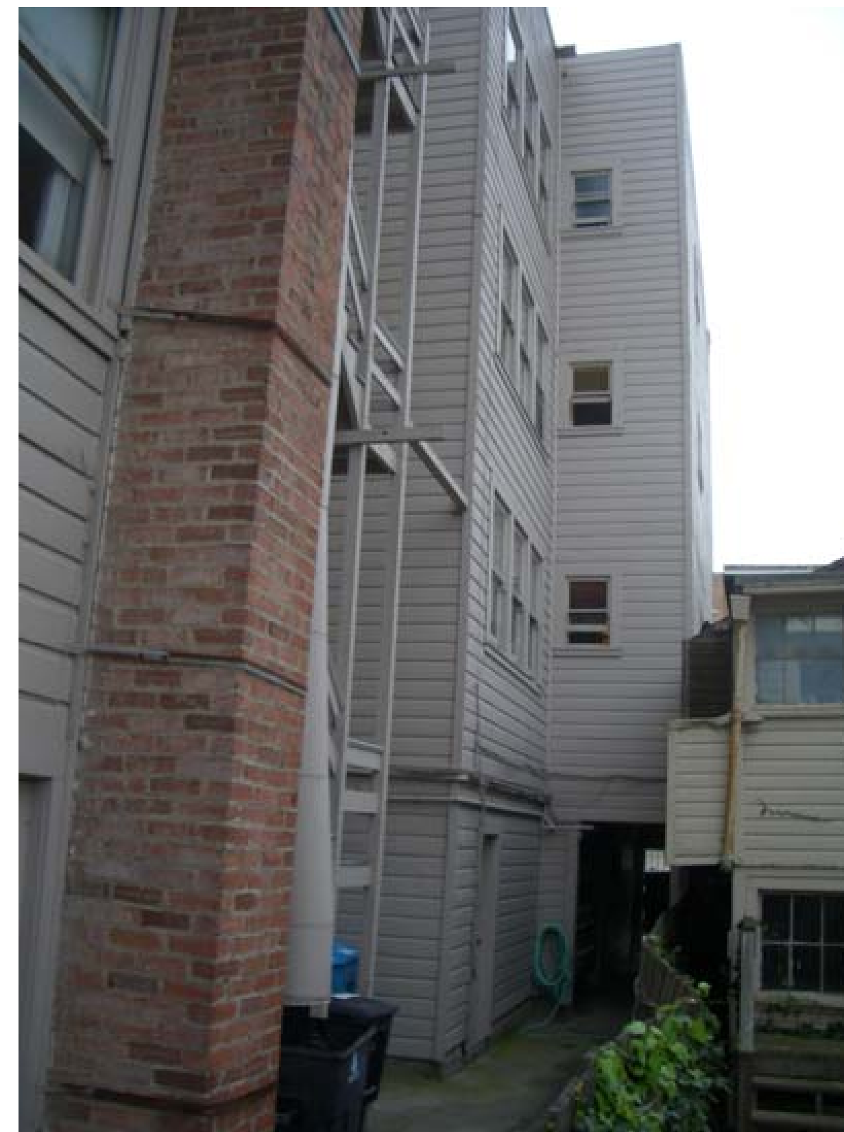
LIGHTWELL AT 1450 CHESTNUT STREET LOOKING SOUTH
