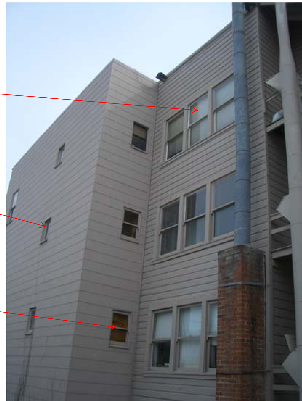
LIGHTWELL AT 1450 CHESTNUT STREET LOOKING NORTH
