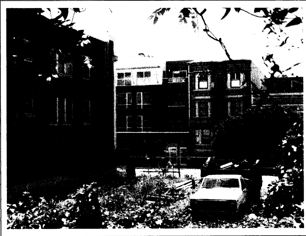
View south from 479 Bartlett - Building abutting east side of project location (3435-3439 26 th st.) burned on 12/21/09.
