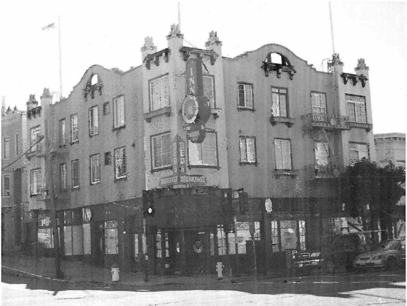
View 1: Existing building frontage.
