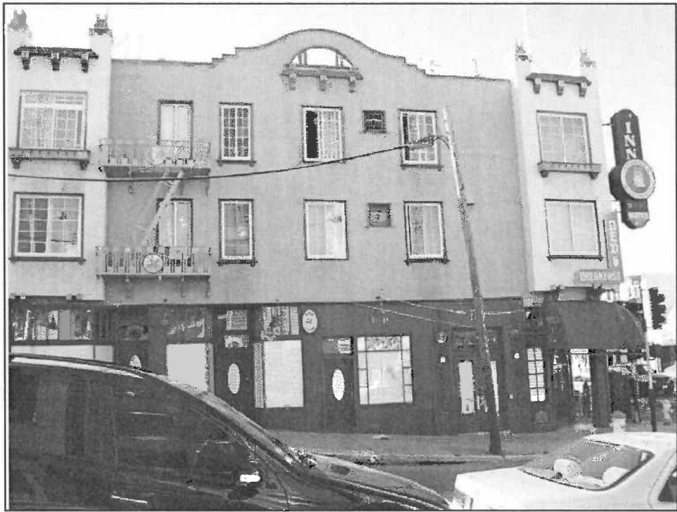
View 3: View to the west of the project building facade on Scott Street.
