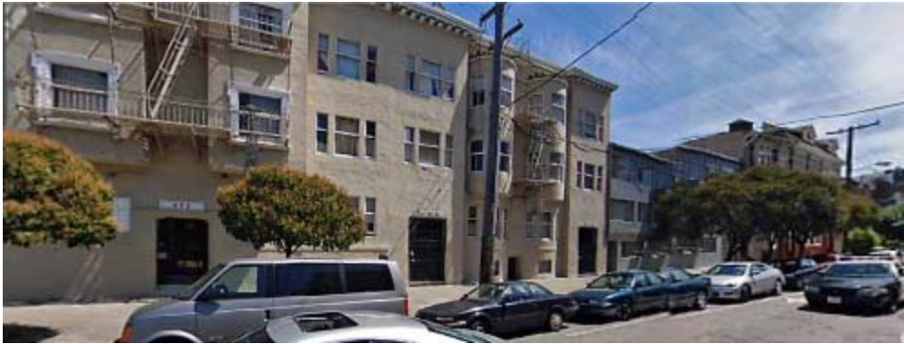
View south from intersection of Baker and Hayes Street
