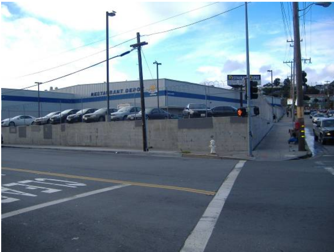
5 - SE corner of building and existing retaining wall - from S side of Napoleon looking North
