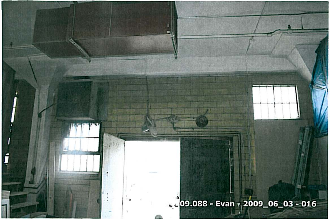
7. Clay Tile Interior Liner of Exterior Wall
