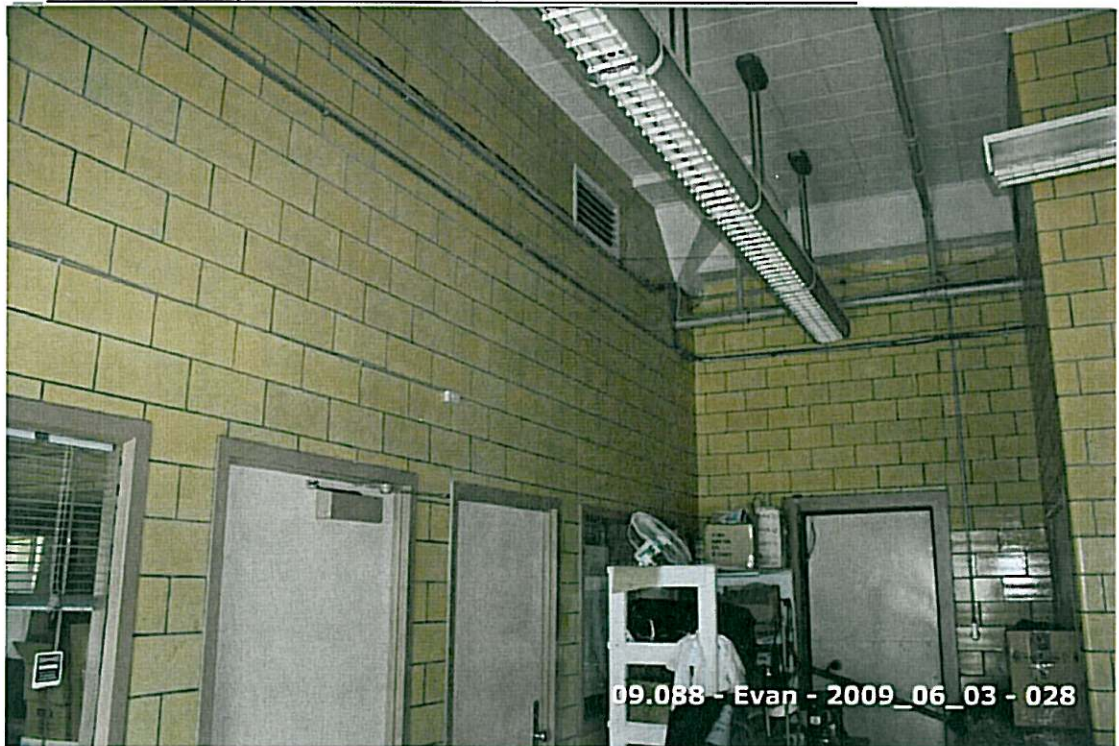
8. Interior Clay Tile Partition
