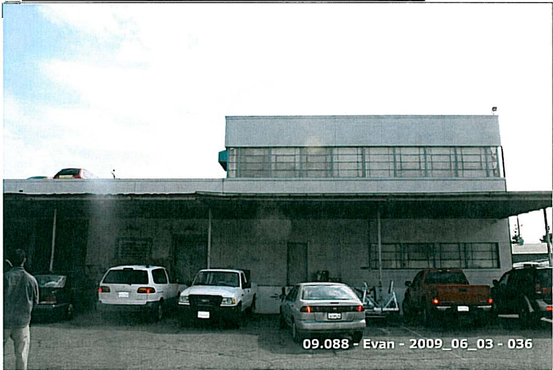
2. West Elevation Showing Loading Dock & 2 nd Story
