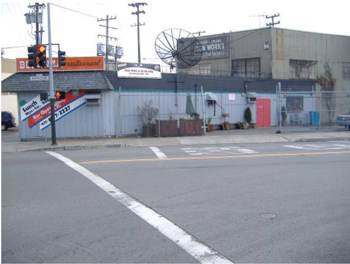
13 - view from Evans & Napoleon intersection looking NW across Napoleon
