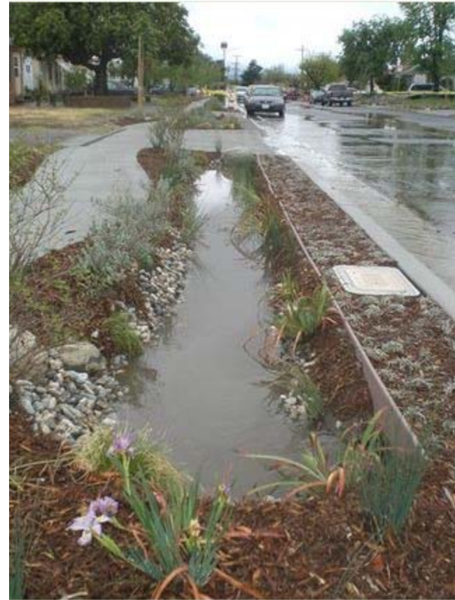
Examples of Installed Bio-Swales
