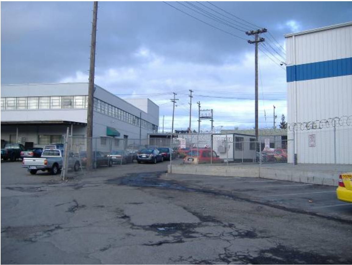
17 - View from center of west property line of the site, looking WNW toward Evans Ave. Power poles to remain, building on left to be demo'd
