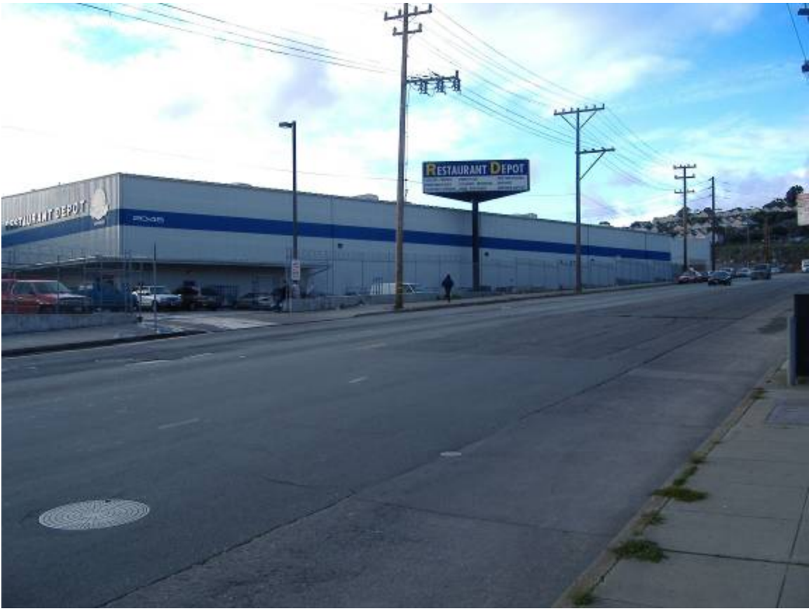
3- Existing building from SE corner of Evans/ Napoleon intersection
