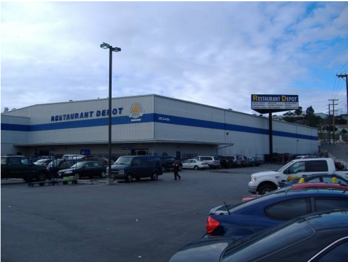
4 - Existing building from SE corner of site
