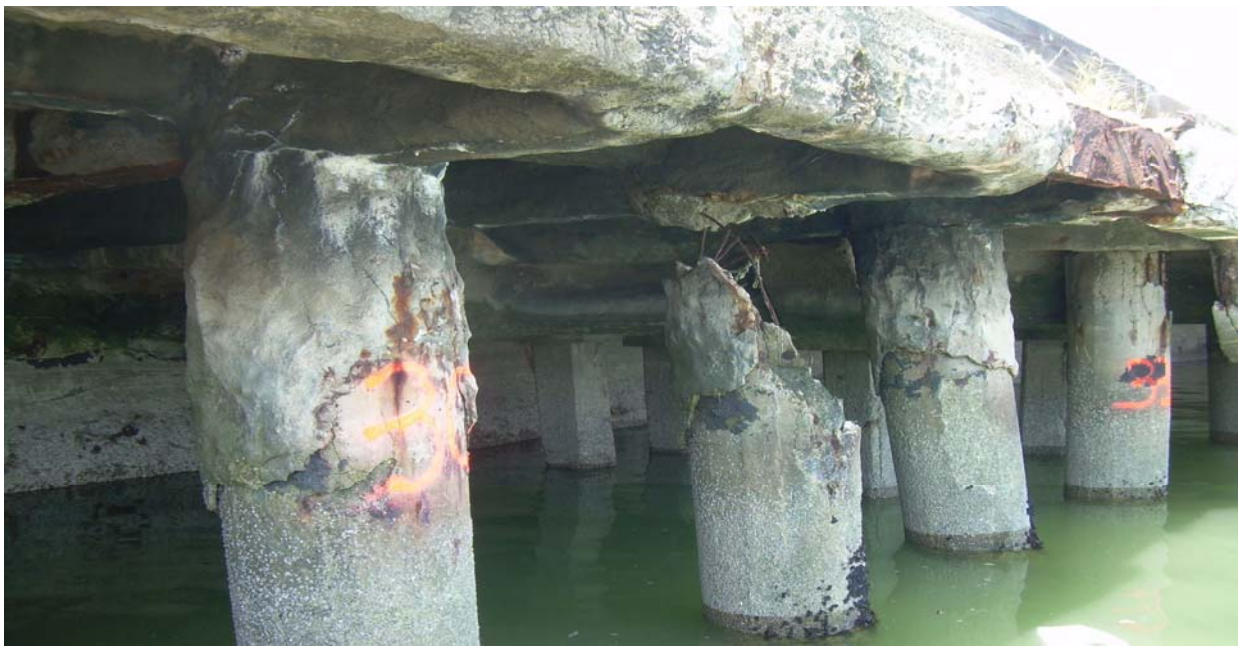
Figure 5 - Existing Bulkhead Wharf Piles and Substructure
