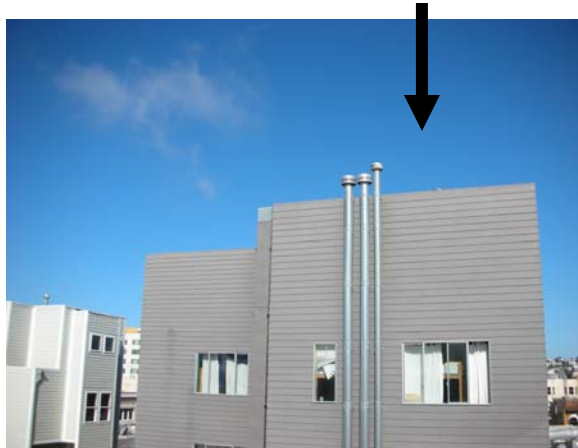
From the Neighbor to the West Looking at Medjool Roof Deck
