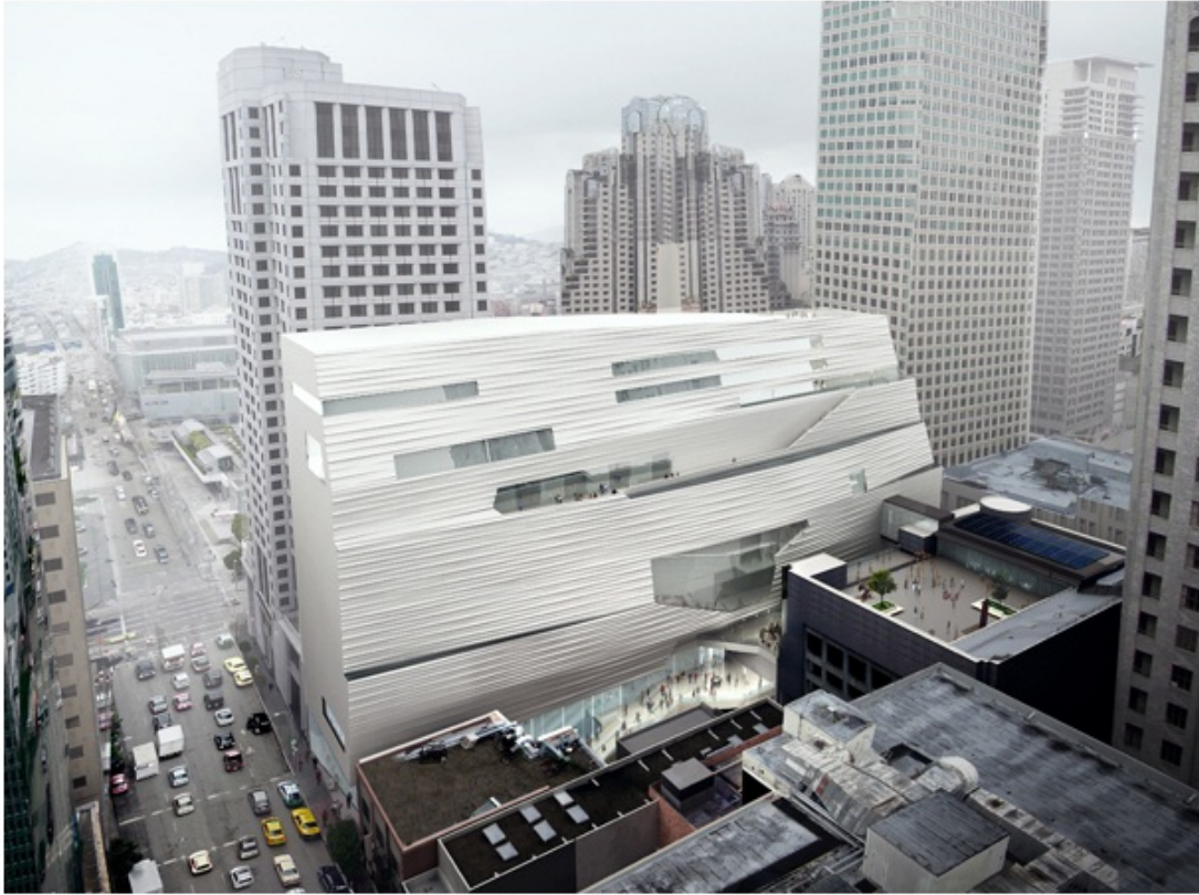
Aerial view of the expansion from Howard Street. Image courtesy Snøhetta.
