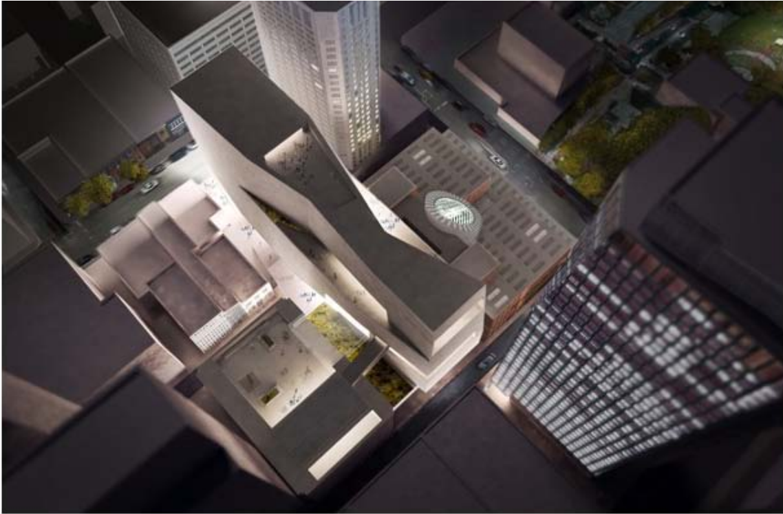
Aerial view of the new expansion from Minna Street. Image courtesy Snøhetta.
