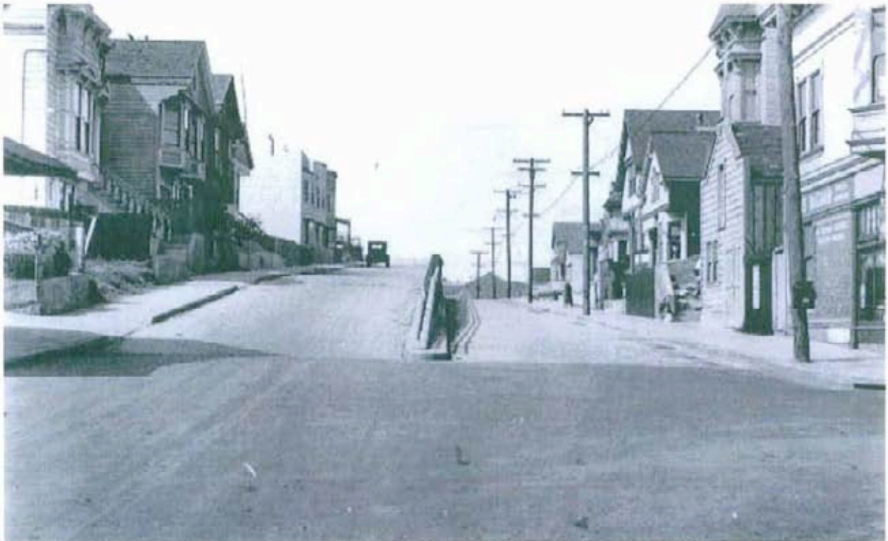
Douglass Street looking northerly from 21 st Street, August 24, 1927. Source: San Francisco Historic Photograph Collection
