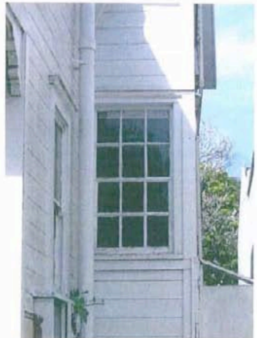
Window on east side
