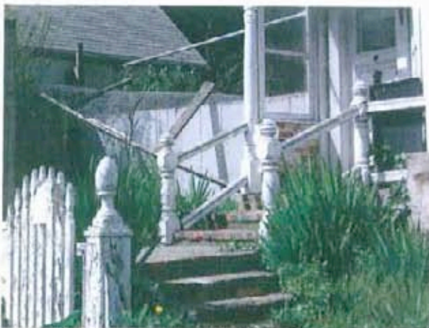
Brick steps and path leading to front entry
