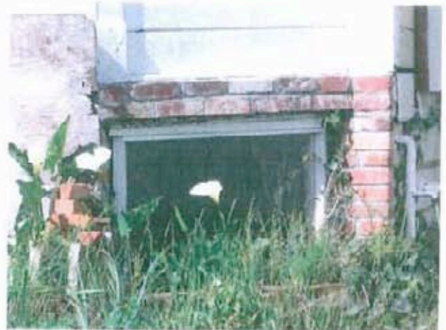
Brick cladding around basement window
