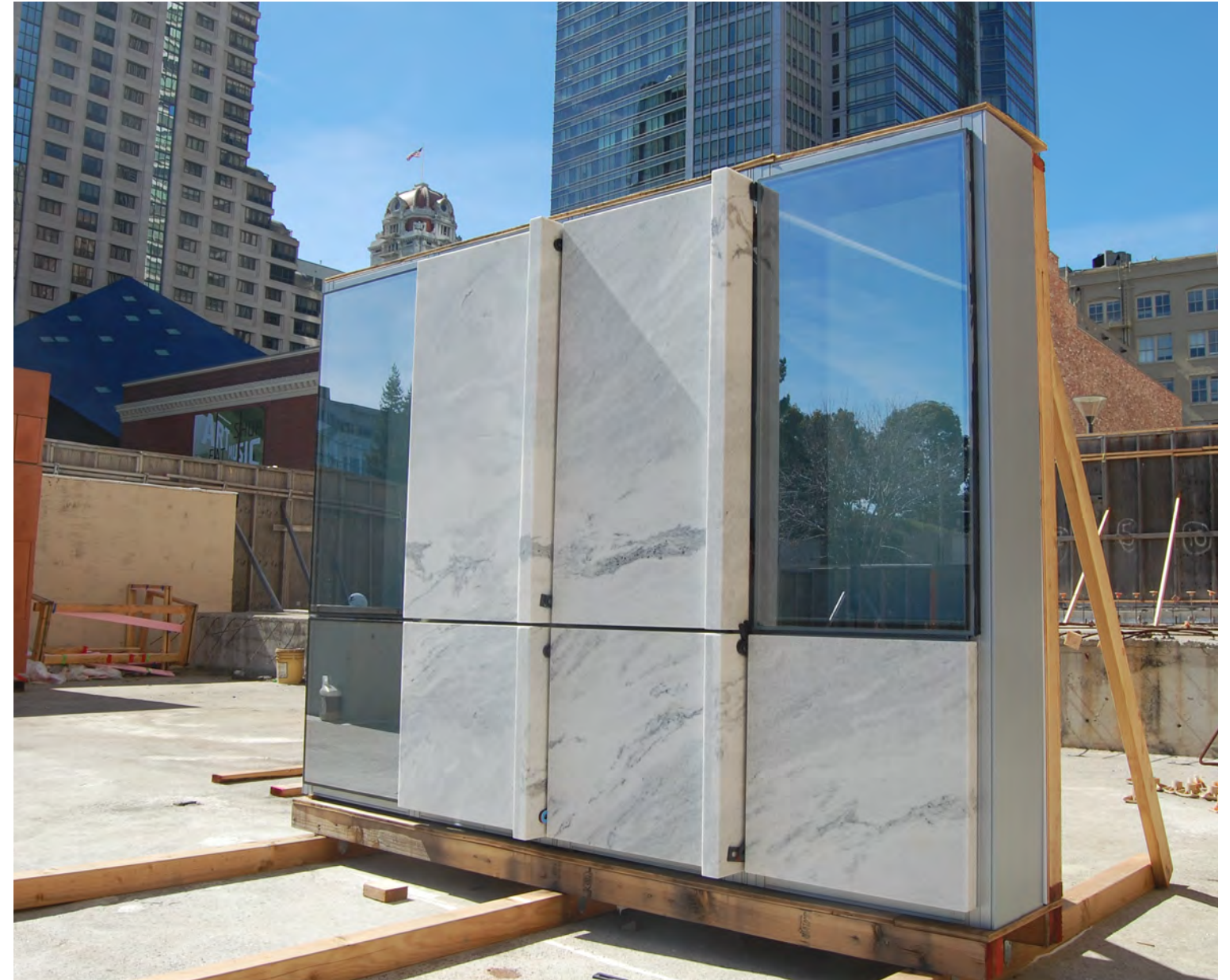
VISUAL MOCK-UP OF TOWER FACADE COMPONENTS
