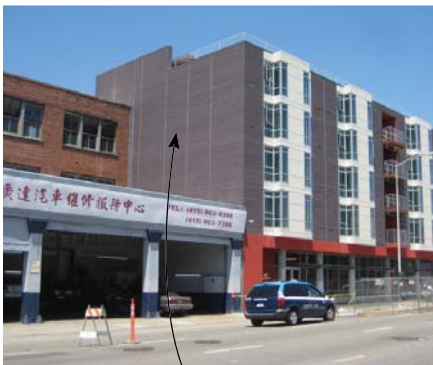
exposed finished building wall
